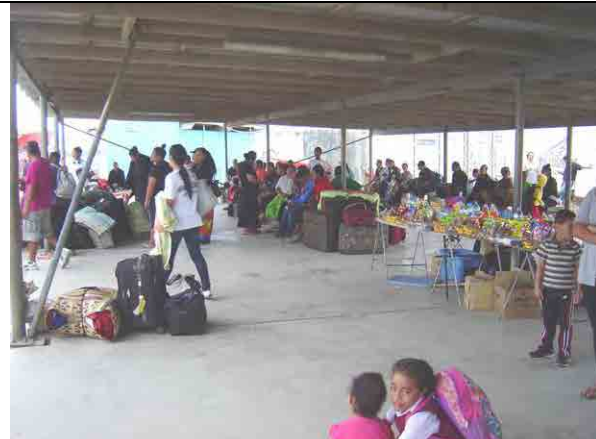
Photo 1-4: Inside of the Waiting Shed There are not enough chairs, and winds and rains blow in. Passengers are suffering severely from sand dust pollution by the strong winds
