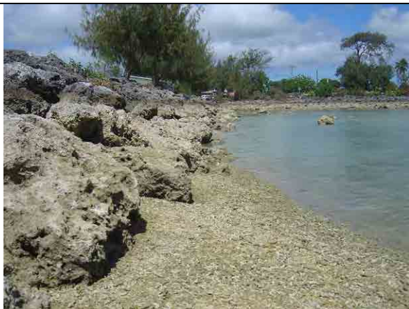
Photo 2-5: Revetment on west side of Faua Wharf
