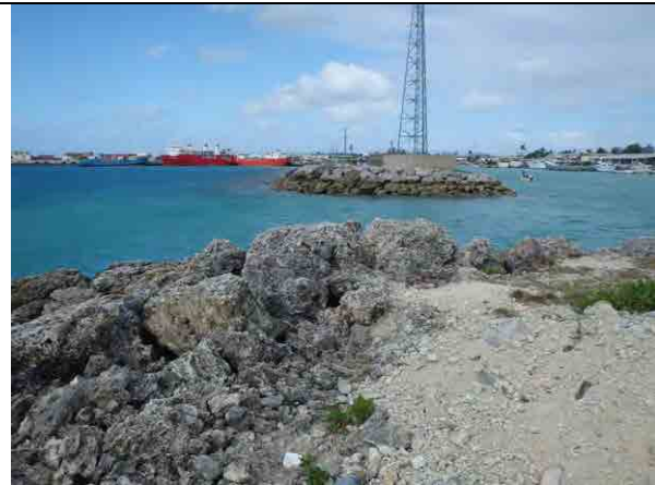
Photo 2-2: Port Entrance at Faua Wharf
