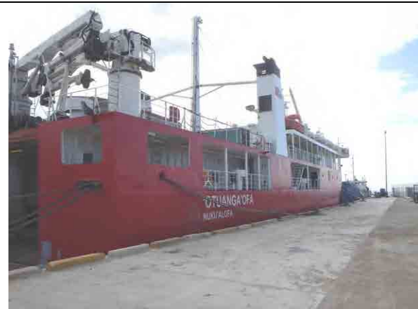
Photo 1-11: MV Otuanga'ofa is mooring at Berth No.3 in Queen Salote Wharf.
