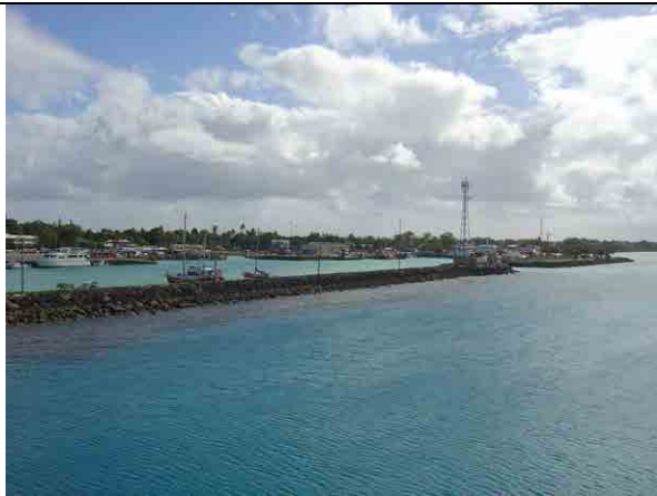
Photo 2-1: Full View of Faua Wharf
