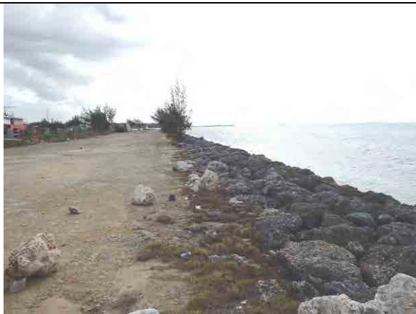
Photo 2-3: Existing Breakwater at Faua Wharf
