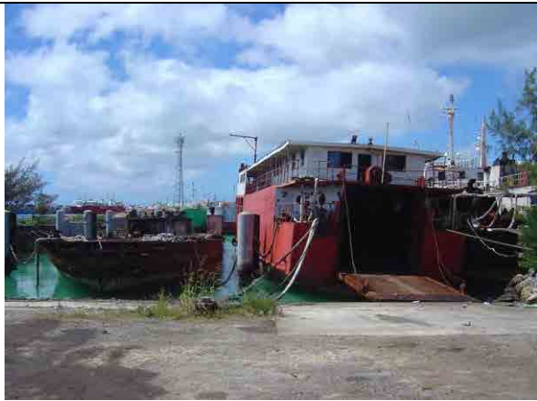
Photo 2-13: West side of Faua Wharf Moored abandoned vessels
