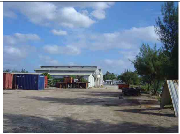
Photo 2-4: East Area of Faua Wharf
