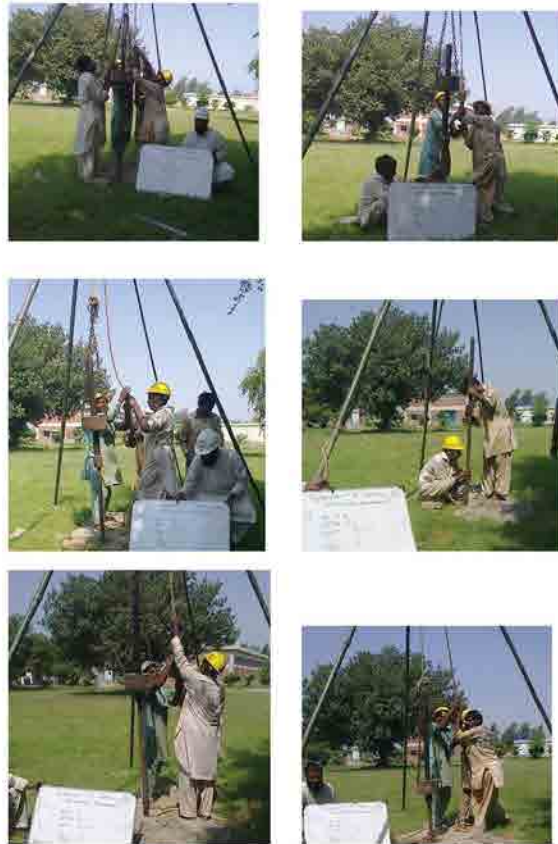
Basin Study - Replacement of Pumping Machinery Faisalabad
