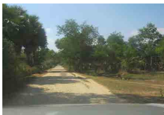
Condition of the road near Labuttalot Village
