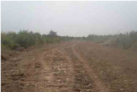
Condition of the road near Meethwaychaung Village
