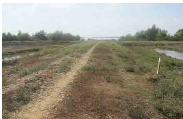
Condition of the road near Labuttalot Village
