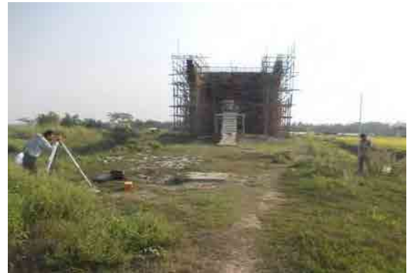
View of GPS Station and Surrounding
