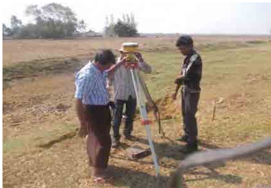
View of GPS Station and Surrounding
