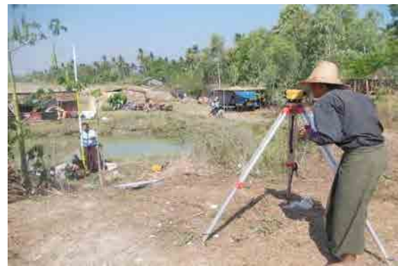
View of GPS Station and Surrounding
