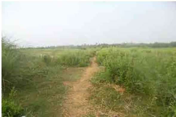
Condition of the road near Kywe Chan Bridge
