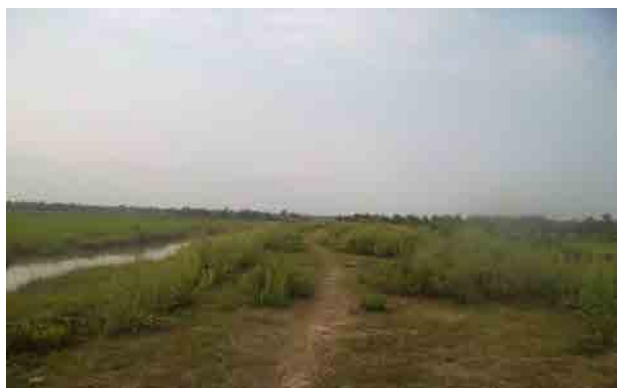
Condition of the road near Kyeechaung Village
