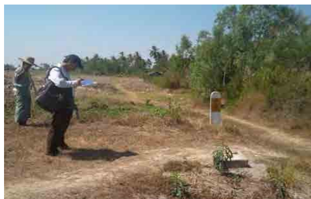
Condition of the road near Ye Tha Phyan village
