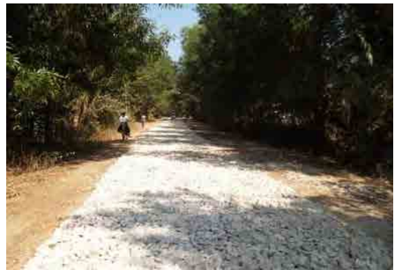
Condition of the road near Satema Village
