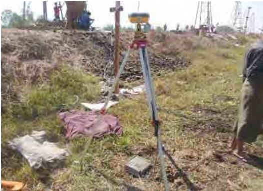
View of GPS Station and Surrounding
