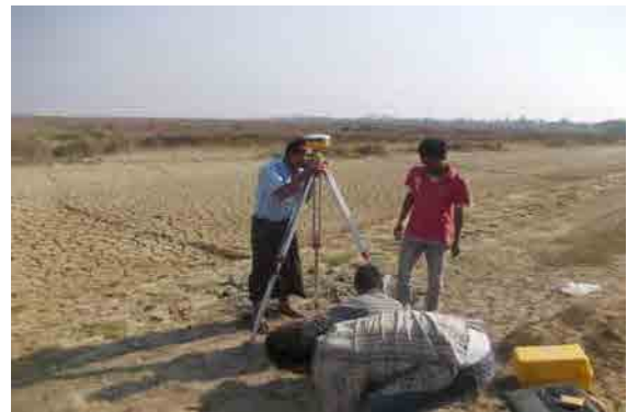
View of GPS Station and Surrounding
