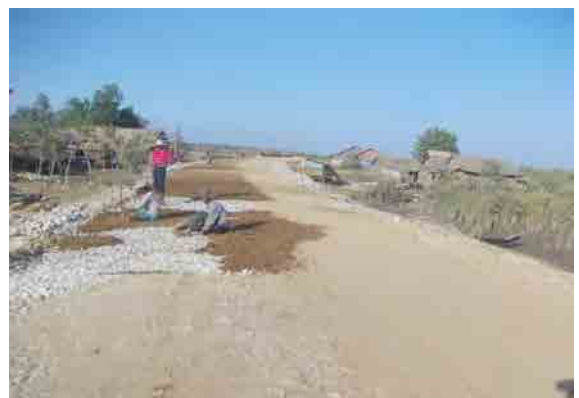
Condition of the road near Lakekwin Village
