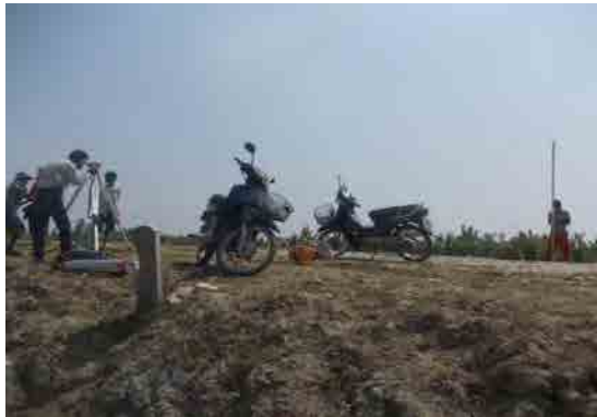
View of GPS Station and Surrounding
