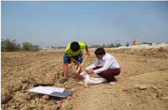
Location-1 (Left bank side of the Bogalay Bridge )
