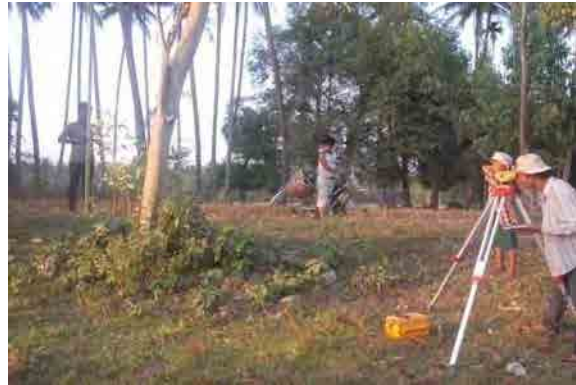
View of GPS Station and Surrounding
