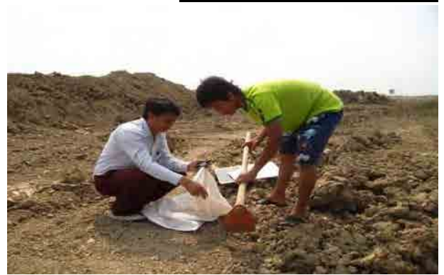
Location-1 (Left bank side of the Bogalay Bridge )
