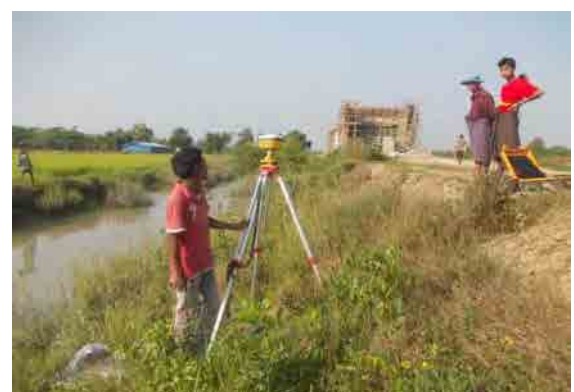
View of GPS Station and Surrounding
