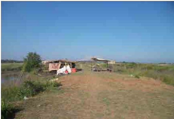
Condition of the road near Pyalate Village
