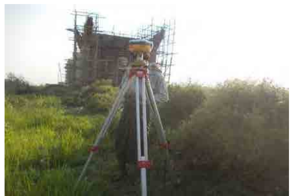
View of GPS Station and Surrounding
