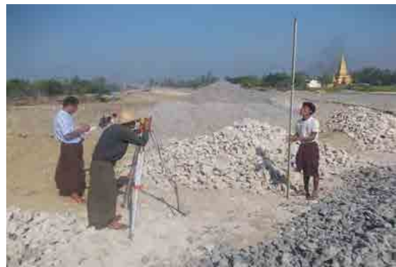
View of GPS Station and Surrounding
