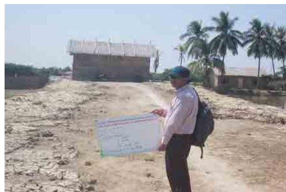
Condition of the road near Salongkya Village
