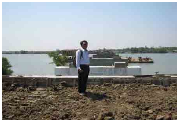
Condition of the road near Chaung-byle-gyi bridge
