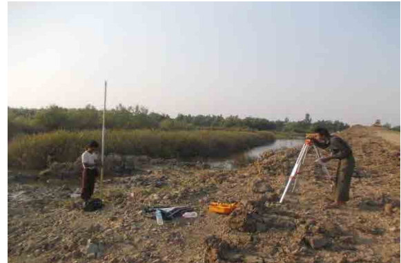
View of GPS Station and Surrounding
