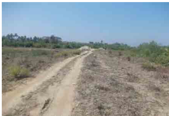
Condition of the road near Ahpyinyesai Village
