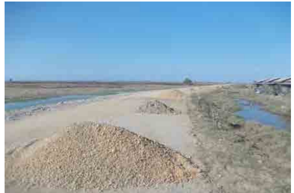
Condition of the road near Tingangyi Village
