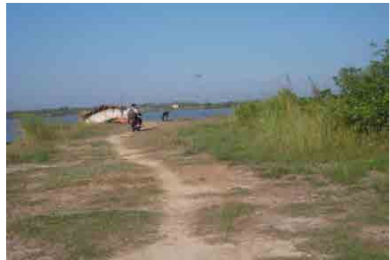
Condition of the road near Ahwachaung Village
