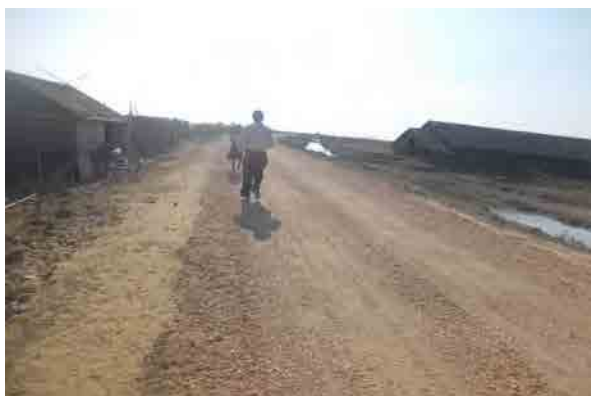
Condition of the road near Kankwin Village
