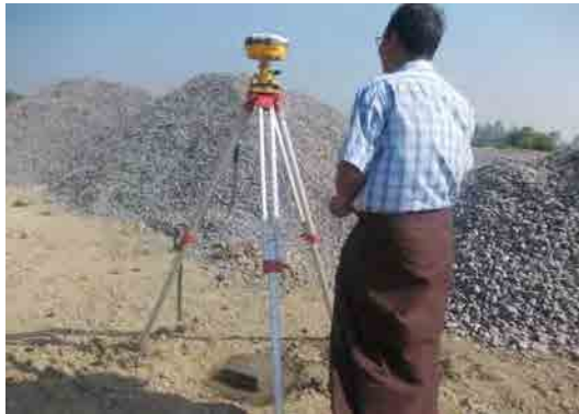
View of GPS Station and Surrounding
