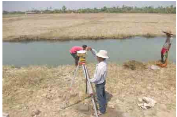
View of GPS Station and Surrounding
