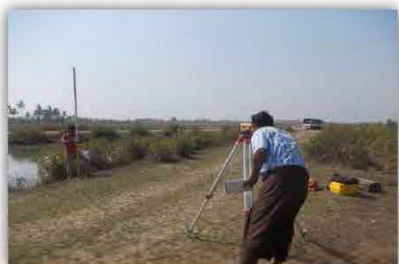
View of GPS Station and Surrounding
