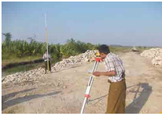
View of GPS Station and Surrounding
