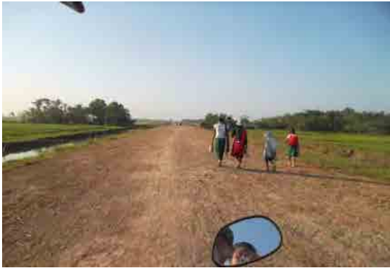
Condition of the road near Mawlamyine-gym
