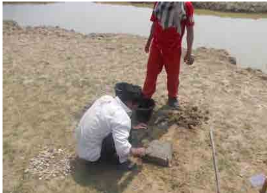
View of GPS Station and Surrounding
