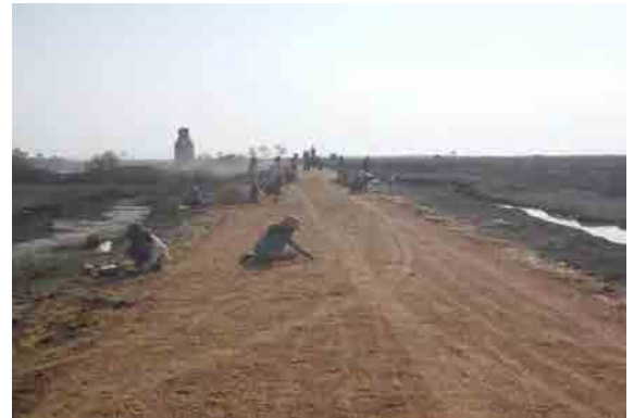
Condition of the road near Thinpoundkwin Village
