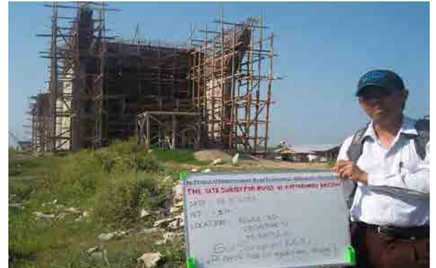
Location-2 (Left bank side of the Kywe Chan Birdge)
