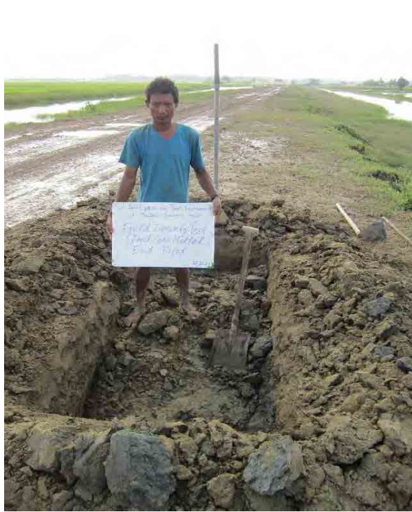
Excavation for Field Density Test
