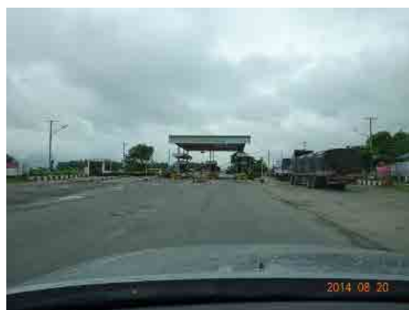
Ph.86 Toll gate (Contractor: ASIA World).
