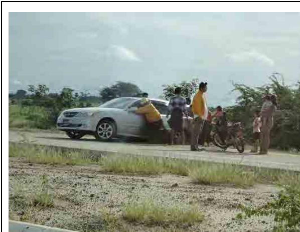
Ph.35 Car could not return to the carriageway by itself due to big gap with the shoulder.
