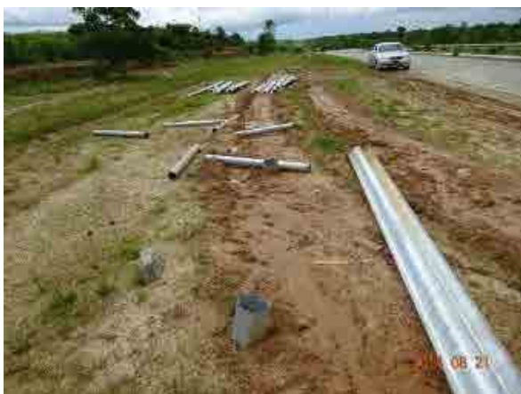
Ph.109 Work site of guardrail installation.
