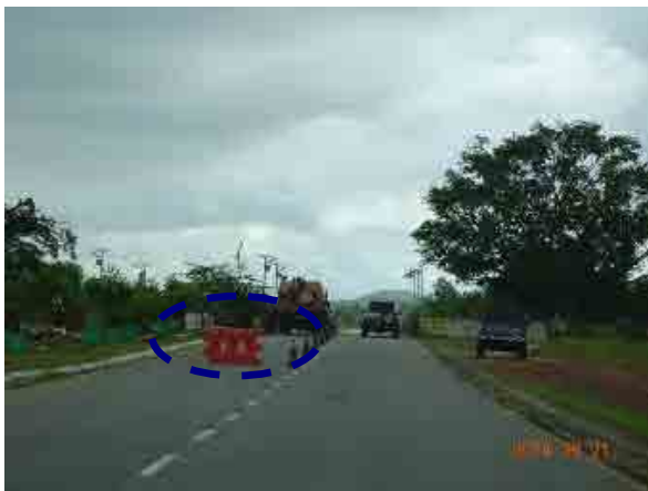
Ph.107 Traffic controlled area should be gradually guided by taper shape.
