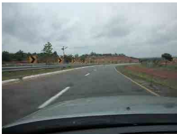
Ph.65 Traffic signs guide the driver's vision in the curve section (good example).
