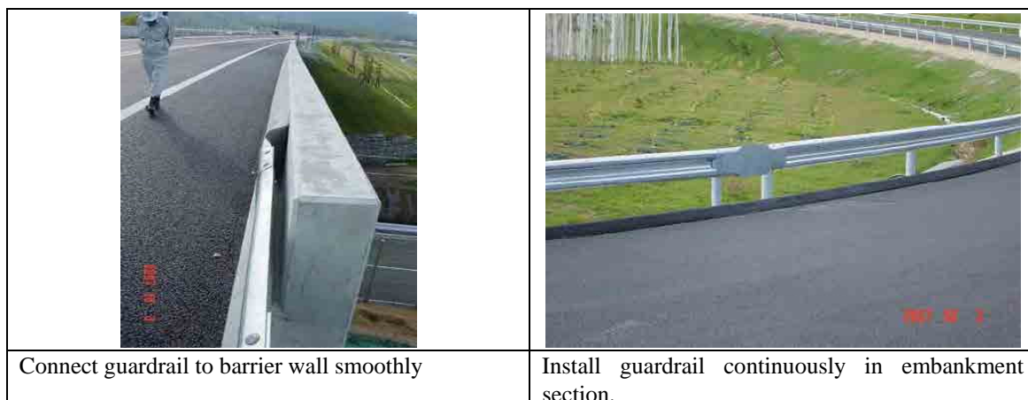
Figure 3.2.6 Arrangement View of Traffic safety Facilities (2)
