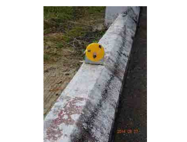
Ph.138 Dust proofing type delineator on curb stone.
