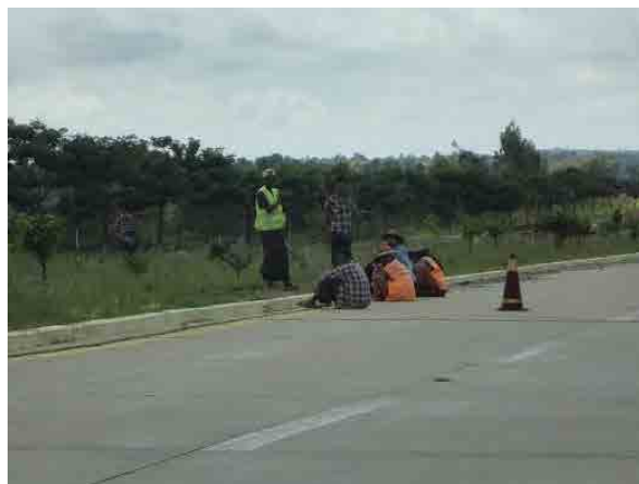
Ph.37 Workers took a rest within carriageway (prohibited work manner).
