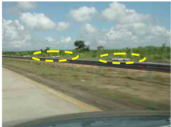
Ph.20 Posts were replaced with guardrail (good example).
