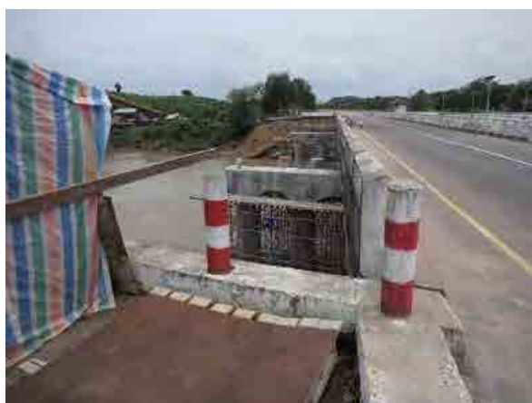
Ph.67 Widening work of the bridge (2-lanes to 3-lanes).
