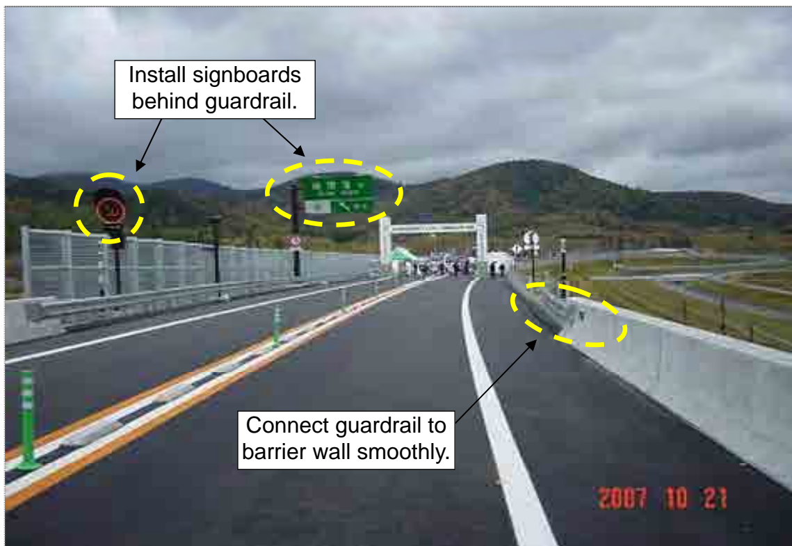
Figure 3.2.5 Arrangement View of Traffic safety Facilities (1)
