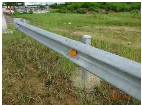
Ph.110 Work site of guardrail installation.
