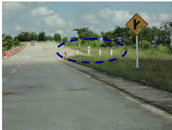
Ph.19 Unnecessary posts should be removed.
