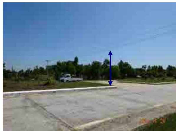
Ph.142 Electric wire seems too low.
