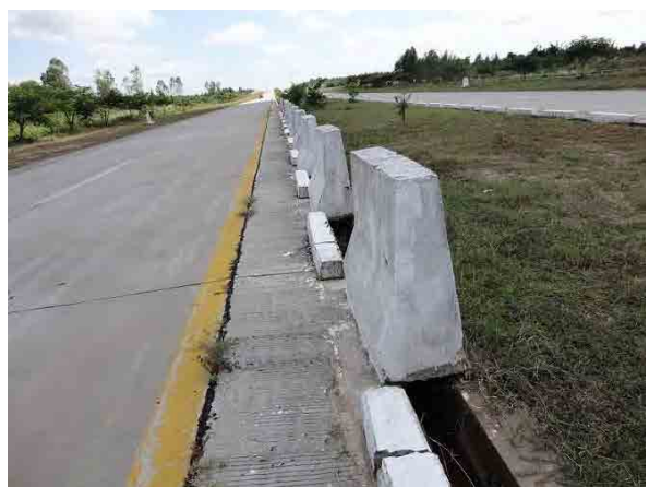
Ph.22 Parapet wall is located behind the curbs.
