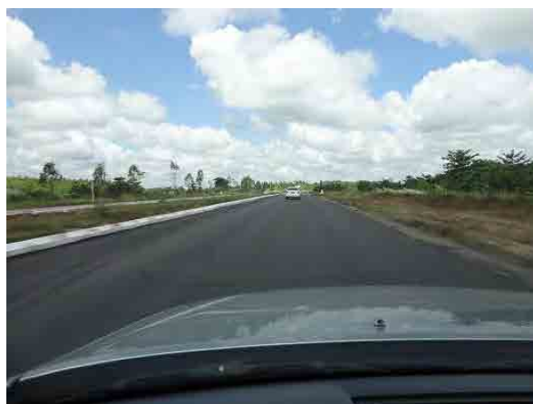
Ph.21 Lane mark should be painted to divide traffic flow clearly.
