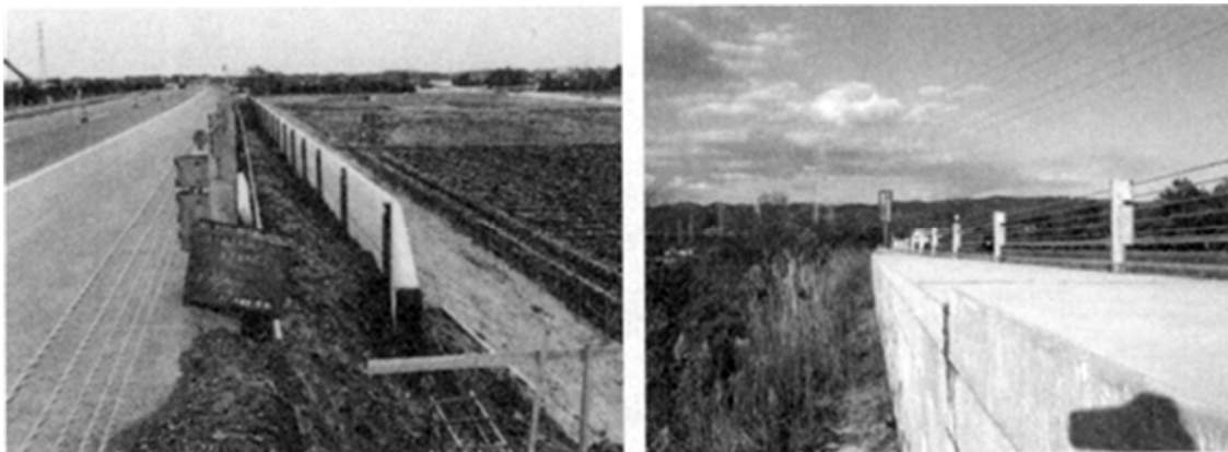
(a) Widening with a retaining wall
