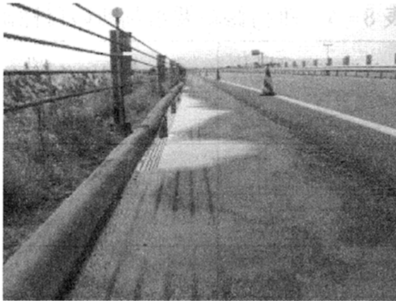
Figure 5-34 Problems due to road surface settlement repair of crash barriers
