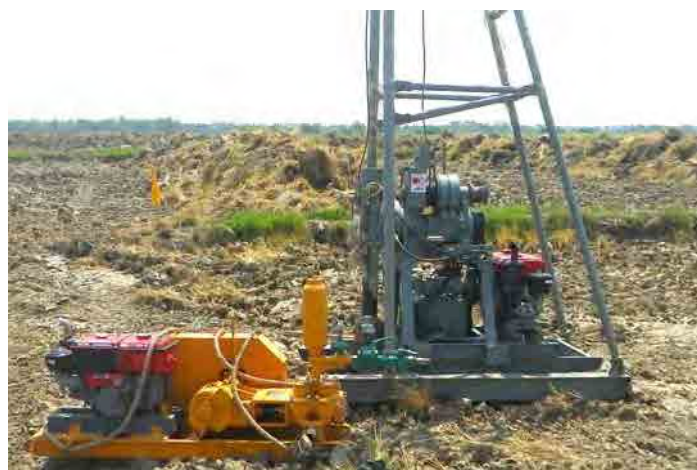
Figure 2-8 Rotary boring machine belong to SRL (TCP)
