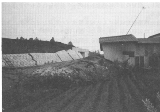
Figure 1-3 Example of slip failure involving the surrounding ground (Japan) 1)
