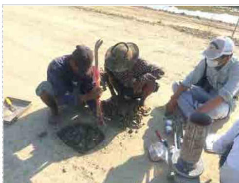
Figure 2.6.3 Work View of FDT (sand replacement method)
