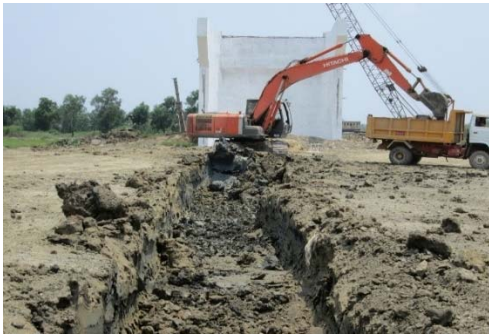
Photo 5 Excavation of Existing road
