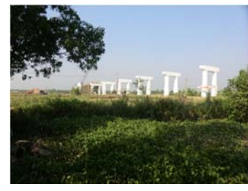
Photo 3 Piers from river side
