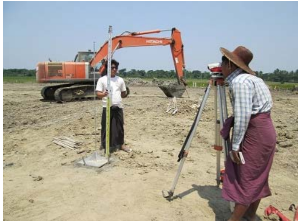
Initial measurement of settlement board after setting at site
