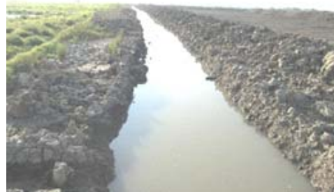
Photo 6 Existed canal along road
