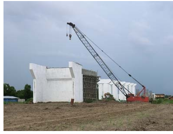
Photo 2 Abutment and piers
