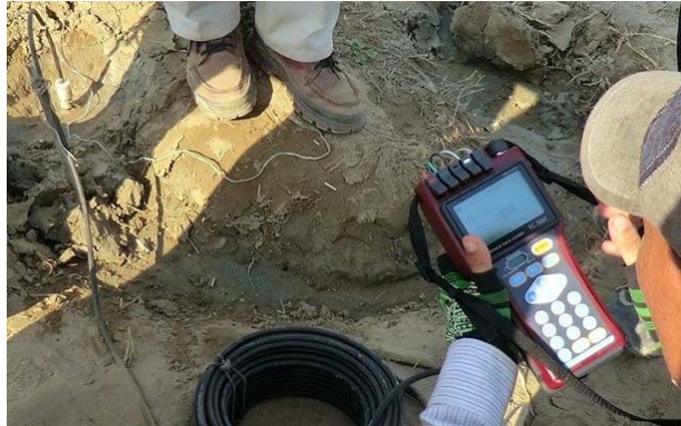
Measuring of Pore Pressure by Data logger
