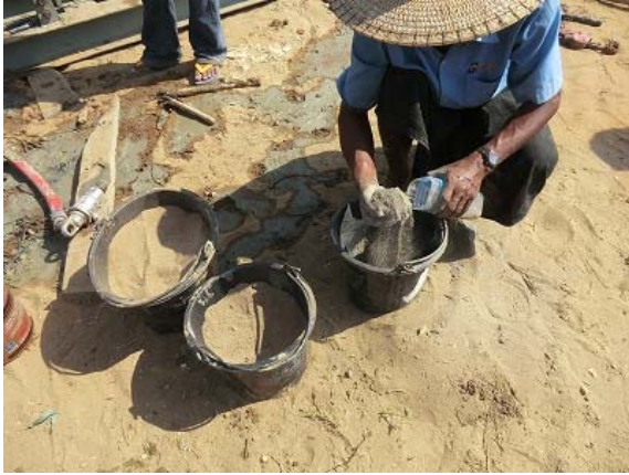
Preparation of Filling materials for bored hole for pore-pressure gauge
