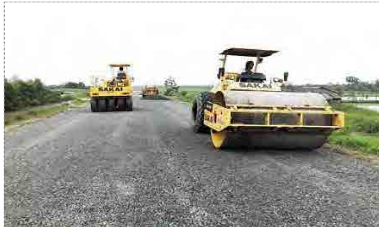
Figure 2.5.9 Work Views of Wearing Course (DBST)
