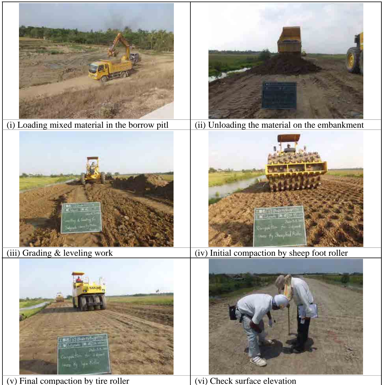
Figure 2.5.5 Work Views of Subgrade Construction
