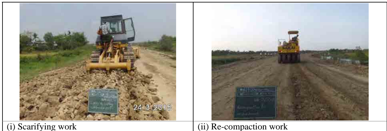
Figure 2.5.2 Work Views of Scarifying and Re-compaction of Existing Embankment
