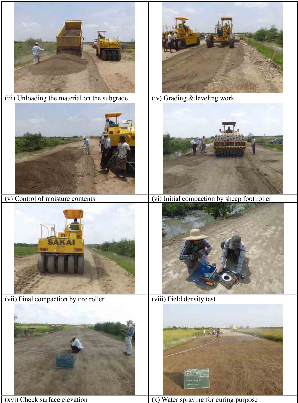
Figure 2.5.6 Work Views of Cement Stabilized Subbase Course Installation
