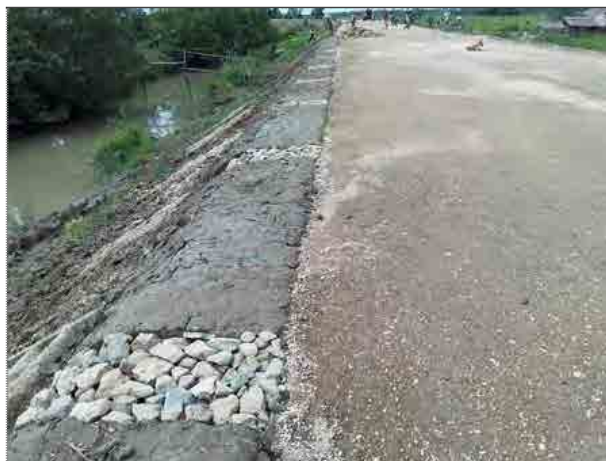
Figure 2.5.11 Work Completion View of Drainage Layer
