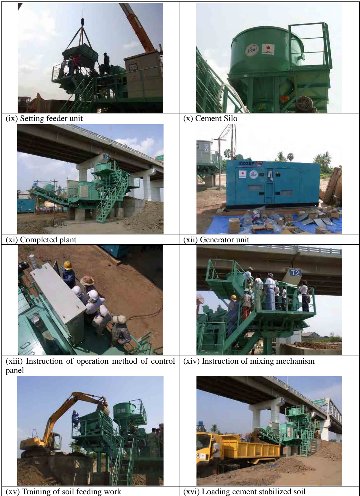
Figure 2.5.1 Work Views of Off-site Work
