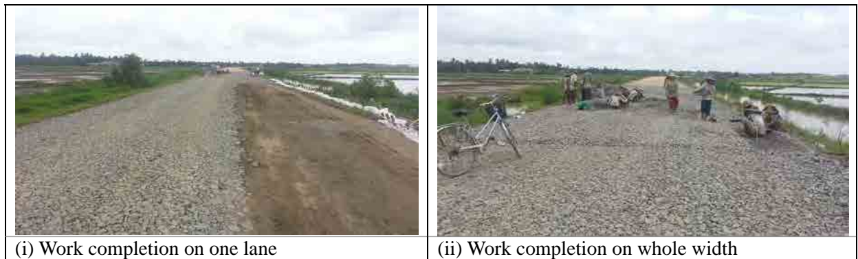
Figure 2.5.7 Work Views of Base Course Installation (Crush Stone)
