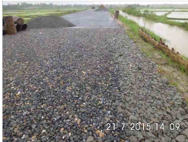
Figure 2.5.10 Work Completion View of Hard Shoulder
