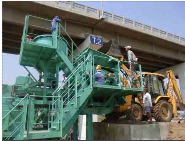
Figure 4.2.3 Training for Material Feeding Work
