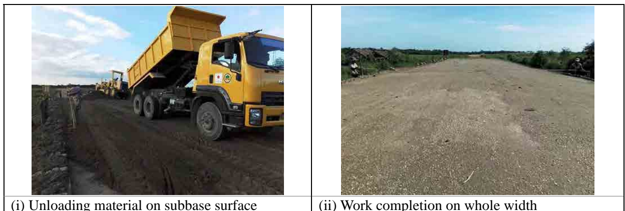
Figure 2.5.8 Work Views of Cement Stabilized Base Course Installation
