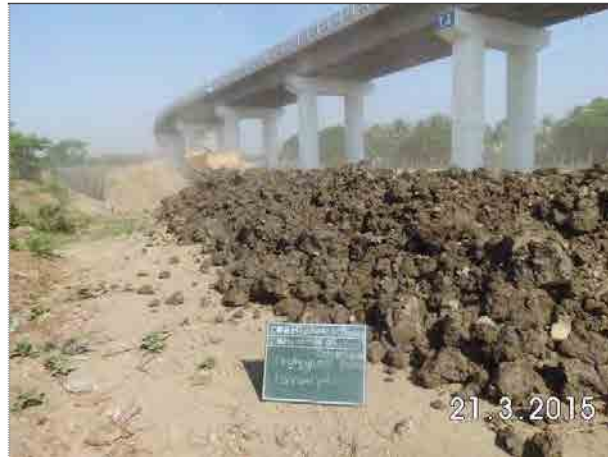
Figure 4.2.4 Soil Drying Work in Yard
