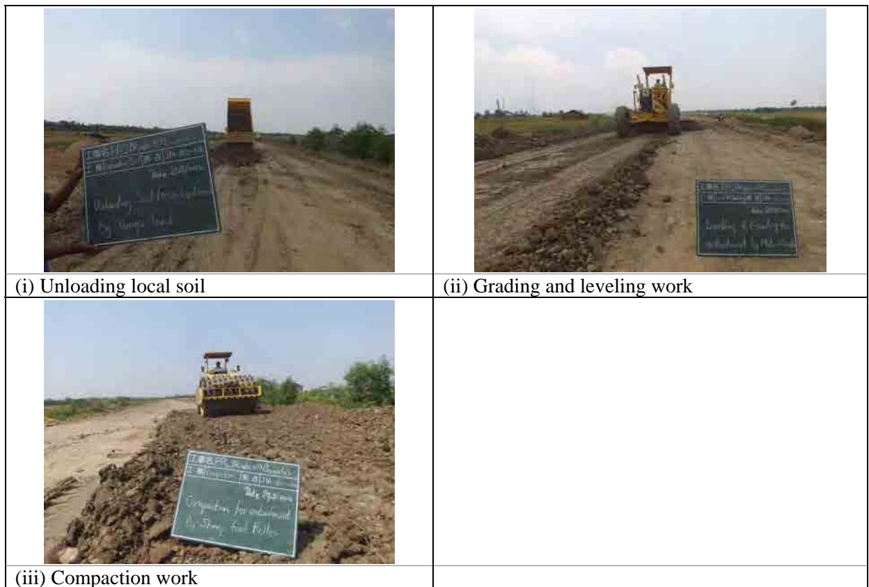
Figure 2.5.3 Work Views of Widening work of the Embankment
