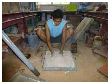
Mixing of materials for stabilization work
