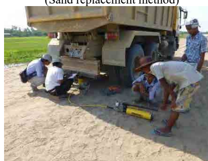
Field CBR test (Plate loading test)
