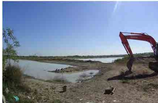
Water condition in Dec 2014 at Borrow pit
