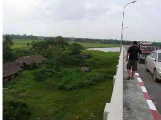
Temporary yard for PP-2 beside Bogaley Bridge
