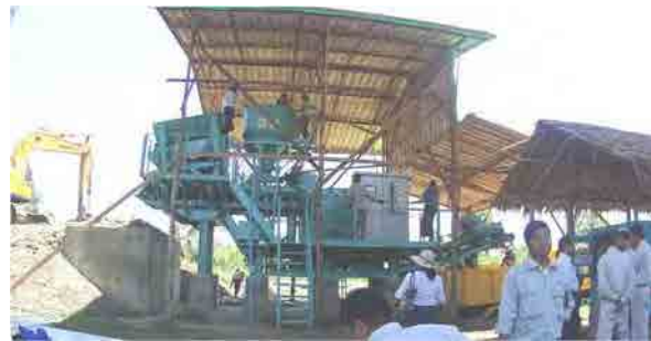
Photo2: Soil mixing plant
