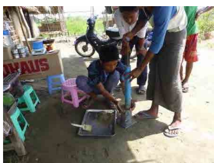
Compaction test on mixing soil in situ
