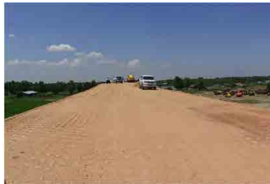
Ditto on Apr 29 2015 (after embankment)
