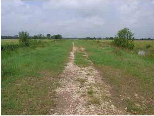
PP-2 実施箇所現況 (Pyapon District, Bogale)
