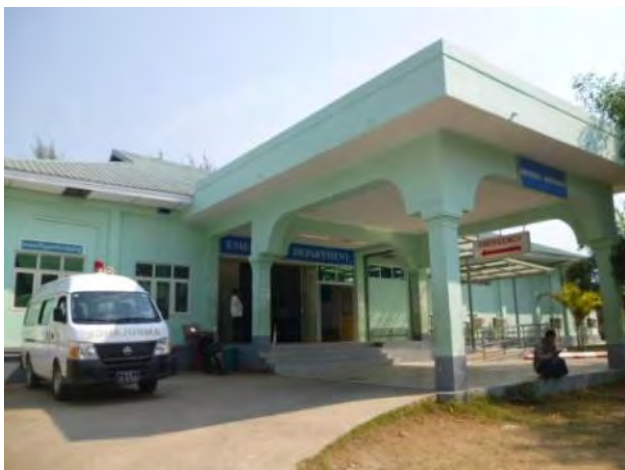
NPT General Hospital Emergency Department
