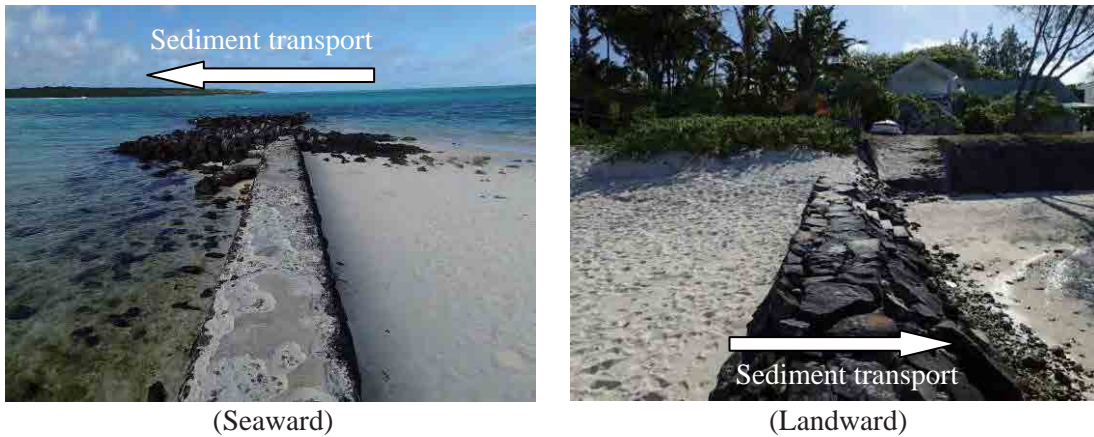
Figure 1.1.2 Beach Profiles across the Groyne at Pte. d'Esny
