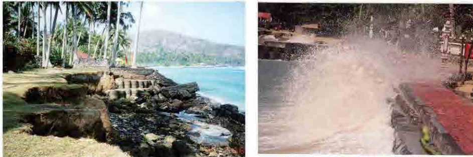
Serious Beach Erosion in Bali
