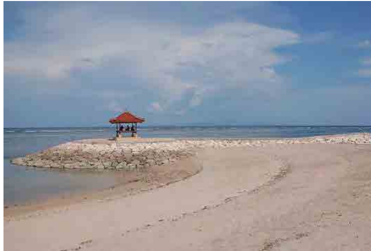
Figure 3.2.6 Example of Well-Environmental Harmonized Groyne (Bali Beach Conservation Project in Indonesia)
