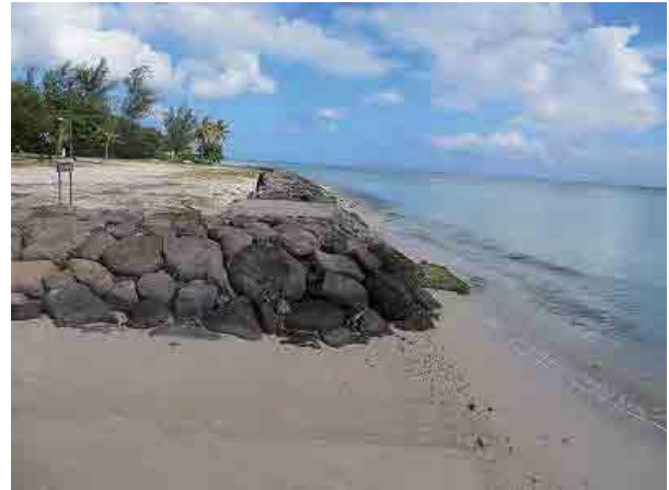
Point F (New revetment on public beach)
