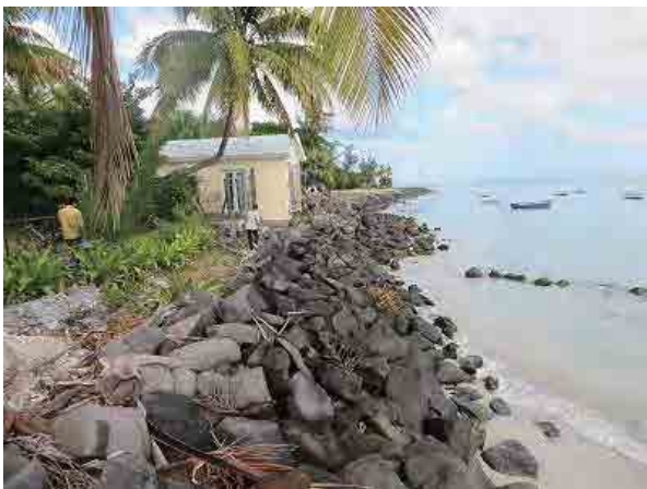
Point E (Boulder protection, approx. 100m east from new revetment)
