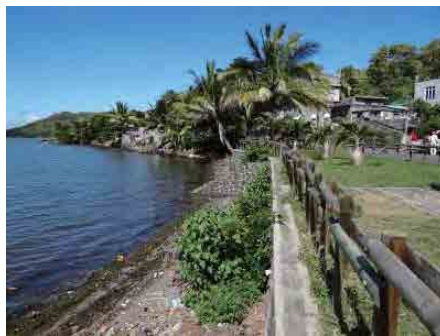
Location 1: Road elevation MSL+2.0m
