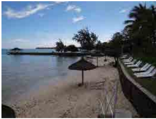
Point A (Groyne in front of the hotel at south area)
