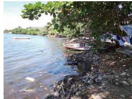
Location 2: Road Elevation MSL+1.6m
