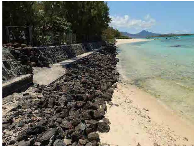
Figure 7.4.12 Existing revetment at Retreat Area in Zone 3
