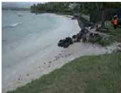
Photo A : Eroded Beach at the West of East Headland in June 2012
