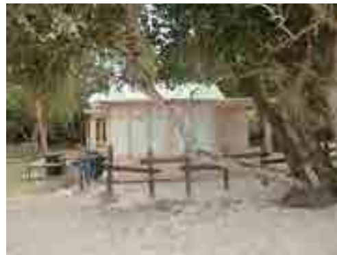
Photo D: Public Toilet
