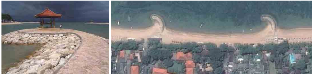
Figure 7.4.11 Image of Curvature Type of Groyne (Case of Beach Conservation Project in Bali, Indonesia)
