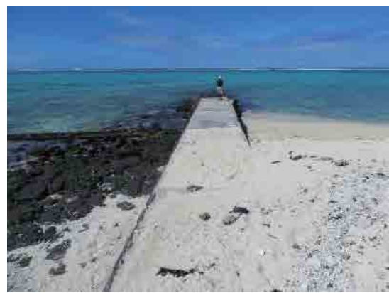
Point B (groyne G1)
