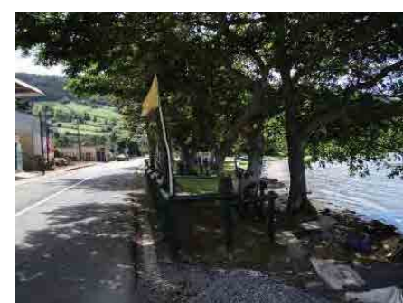
Location 4: Road Elevation MSL+2.4m
