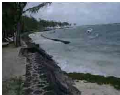
Photo B : Revetment and Detached Breakwater on front of the East Hotel in June 2012
