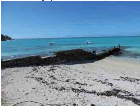
Point C (groyne G2)
