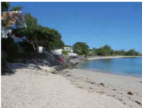
Point E (Eroded area, looking to the west)
