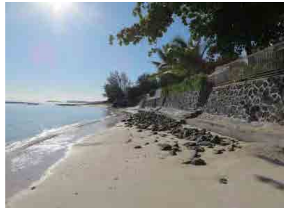
Point D (Eroded area, looking to the east)
