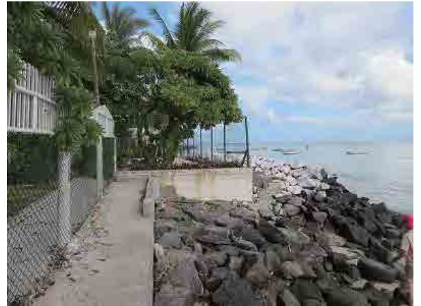
Point D (Boulder protection, approx. 100m east from new revetment)
