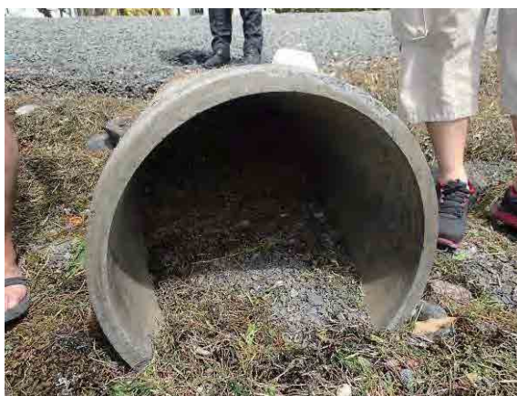
Figure 8.3.33 Condition of Outlet of Drainage Pipe
