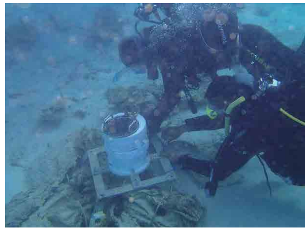
(Item 1-2) Installation of wave current meter
