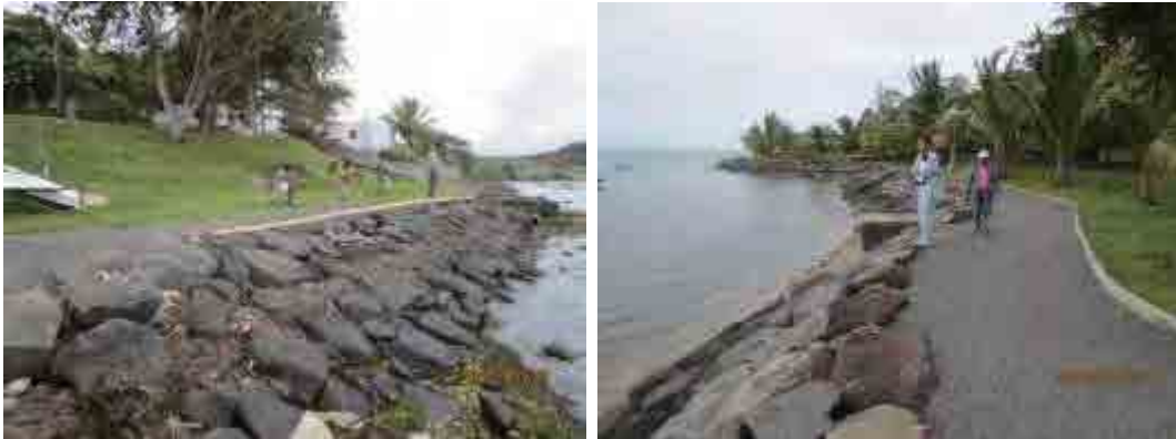
Figure 2.4.5 Rock Revetment in the South of Grand Sable
