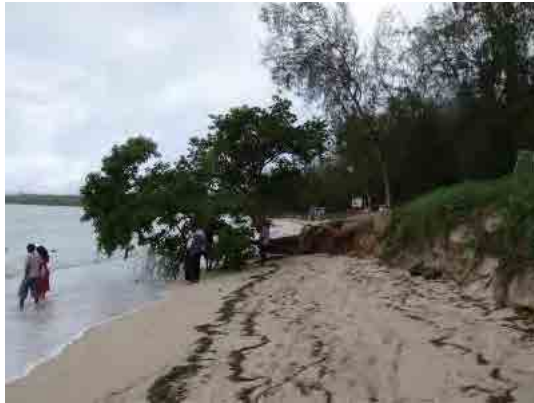
Beach scarp at the upstream side
