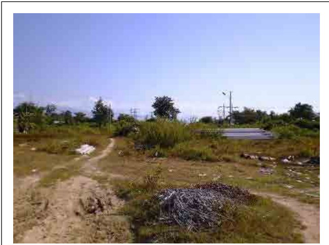
New Bhamo S/S Construction Site
