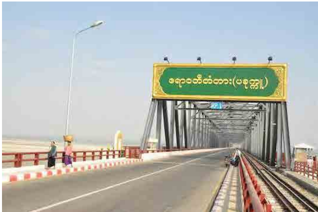
Pakokku Bridge over Ayeyarwady River
