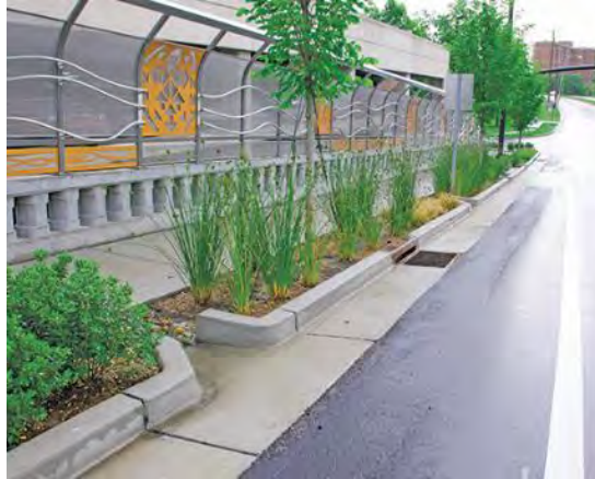
Figure C-2 Example of Bio-retention Planting Strip
