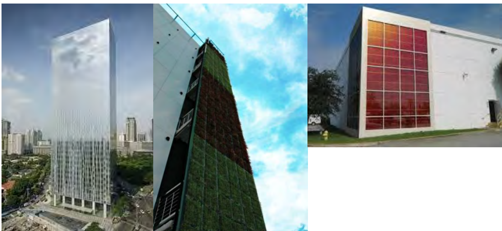
Figure 3 Use of Energy Efficient Curtain Glass Wall, Green Wall, and Solar Panels
