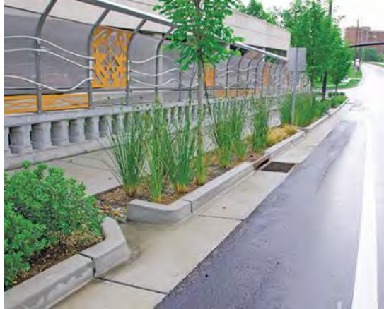
Figure C-2 Example of Bio-retention Planting Strip
