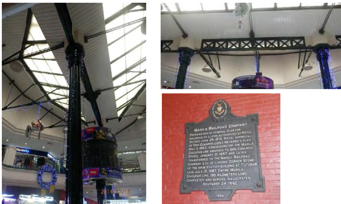
Figure 4.2.5 Original Cast-Iron Columns, Roof Trusses, Beam and Historical Marker
