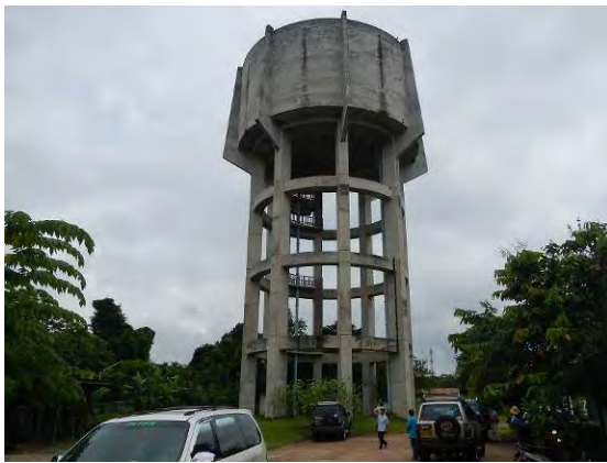
Salakham elevated tank
