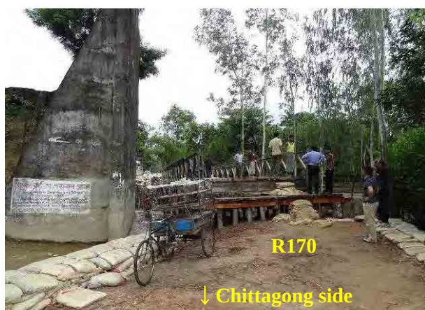
Impassable bridge by car in Upazila Pekua
