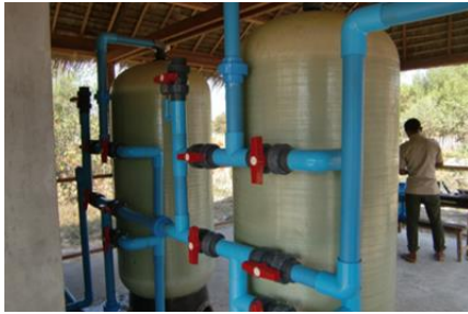
Photo 2-4 Pilot Water Supply System
