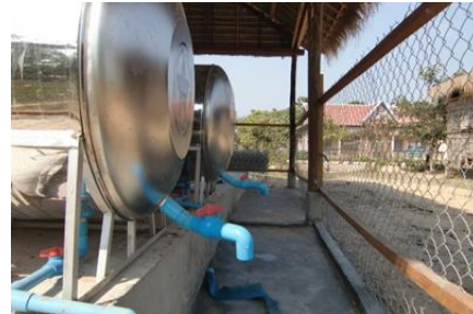
Photo 2-5 Pilot Water Supply System
