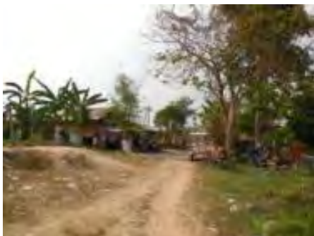
Communities Remaining at Ongoing Container Yard Construction Site (Part 3)
