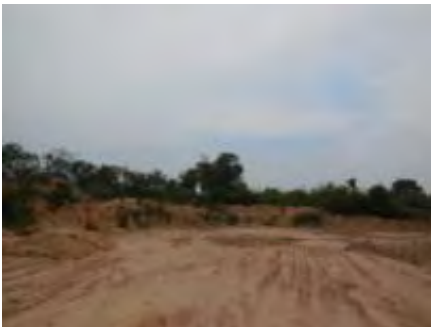
Ongoing Railway Extension Construction Activity at Northern End (Part 1)
