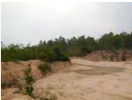
Ongoing Railway Extension Construction Activity at Northern End (Part 3)
