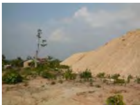
No slope protection at soil dumpsite. Several community houses still exist (Part 1)
