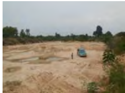
Ongoing Railway Extension Construction Activity at Northern End (Part 2)
