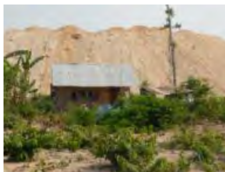
No slope protection at soil dumpsite. Several community houses still exist (Part 2)
