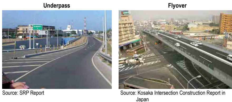
Figure 5.3.4 Examples of Underpass and Flyover
