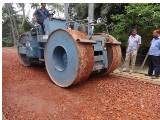
Compaction of brick sub-base
