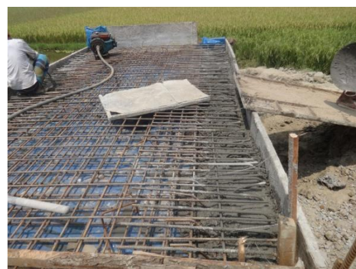
Concrete casting for box culvert
