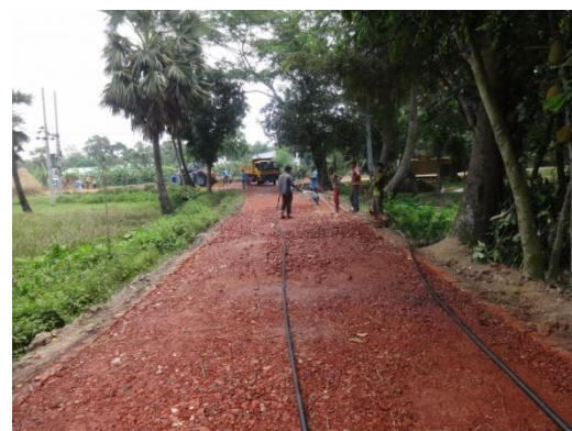
Water spraying for brick sub-base
