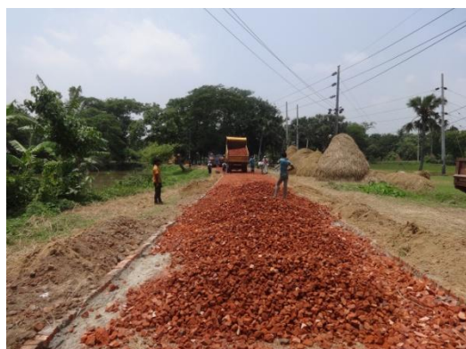
Laying of brick sub-base
