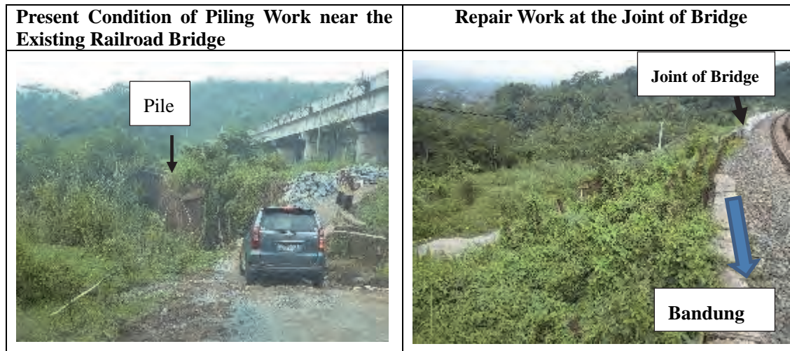
Figure 4.2-9 Condition of Existing Landslide (Sta. 81km)
