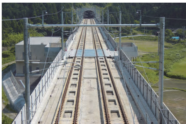
Figure 10.3-1 Framed-shaped Slab on Shinkansen Viaduct
