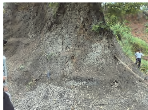
Figure 7.2-10 Condition of Slaking of Mudstone (Jatiluhur formation)
