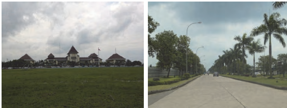
Left: Government Office Complex, Right: Boulevard in the Industrial Park Source: JICA Study Team
