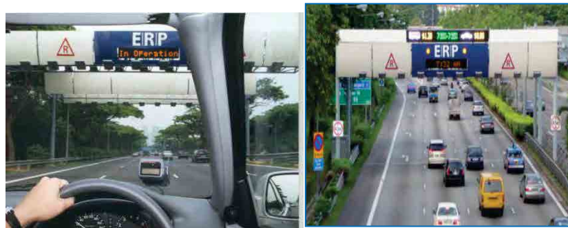
Figure 11 (OBU on windscreen, ERP overhead gantry)
