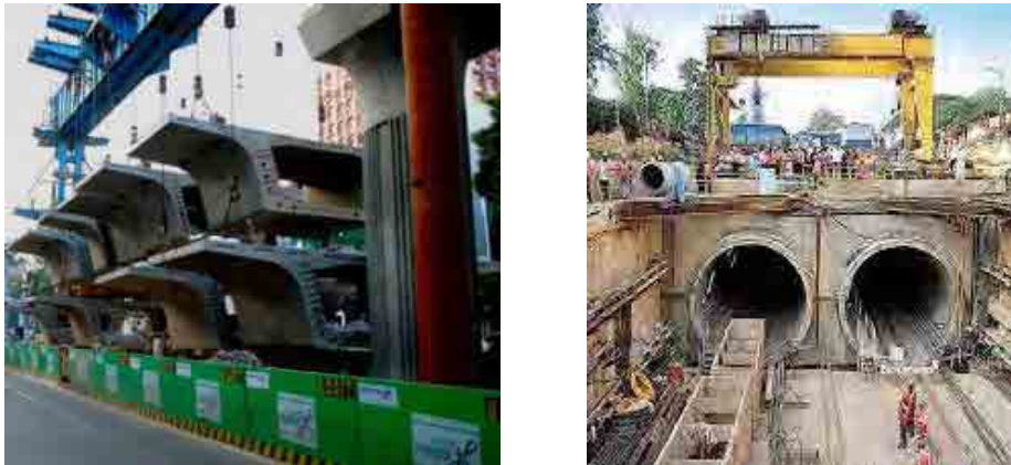
Figure 2.6 Construction Sites of Metro
