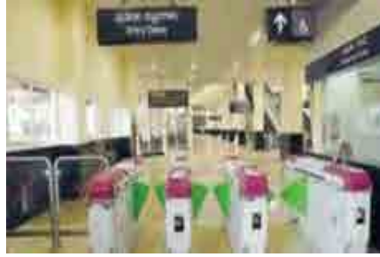
Entry and Exit Gates in Metro
