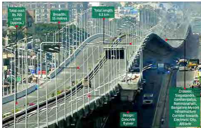
Figure 2.43 Bangalore Elevated Tollway
