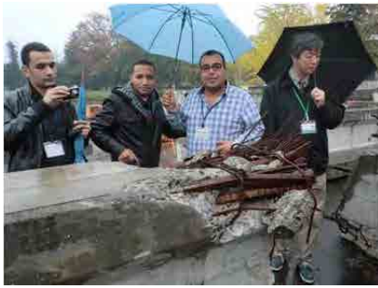
Observation of damaged bridge members at Public Works Research Institute.
