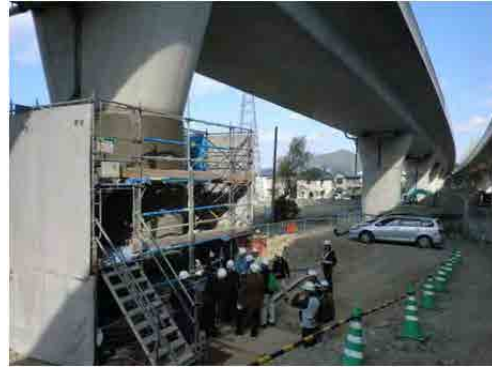
Observation of bridge reinforcement work
