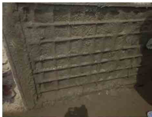
Picture 2-7 OST on shotcrete process
