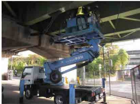
Inspection practice using a bridge inspection vehicle
