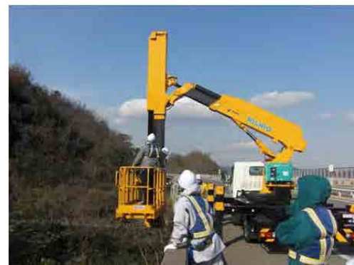
Inspection practice using a bridge inspection vehicle
