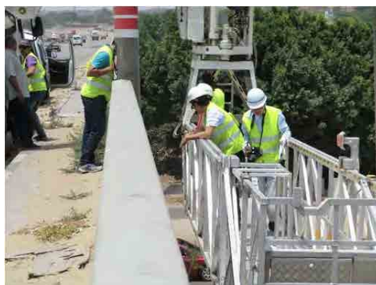
Inspection using BIV
