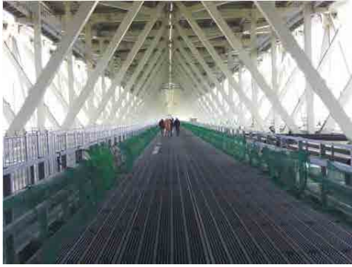
A tour of Akashi Kaikyo Bridge to observe the inspection facilities.
