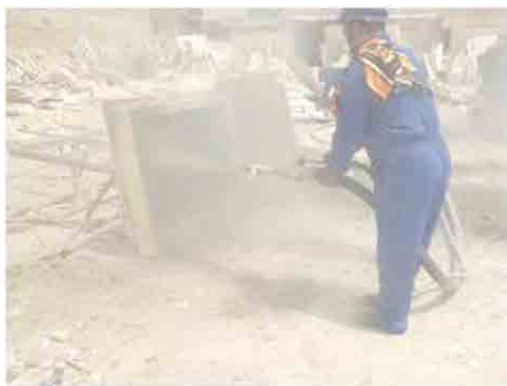
Picture 2-7 OST on shotcrete process
