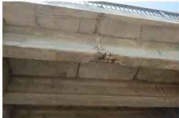
Girder Rebar Corrosion (Bad) Severe corrosion.
