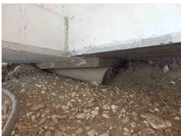
Confirming a bearing that is nearly entirely buried in sand
