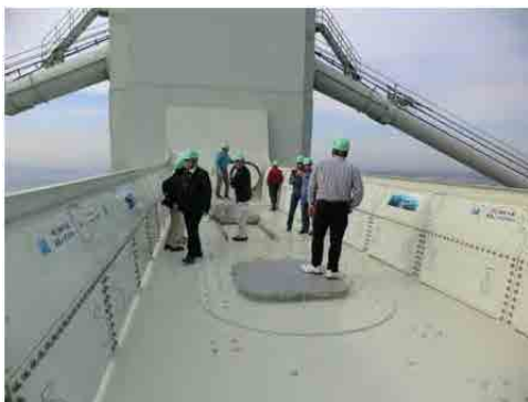
Observation of maintenance facility of Akashi Kaikyo Bridge
