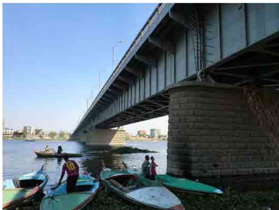
Picture 2-5 Old steel bridge in good condition
