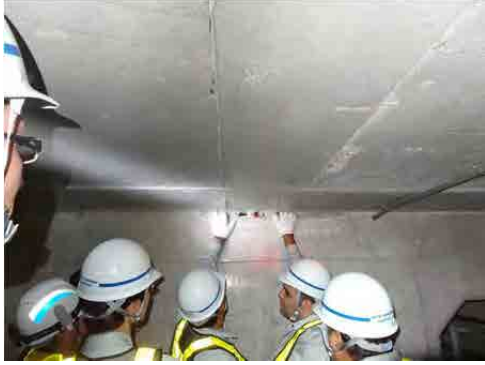
Concrete bridge inspection practice
