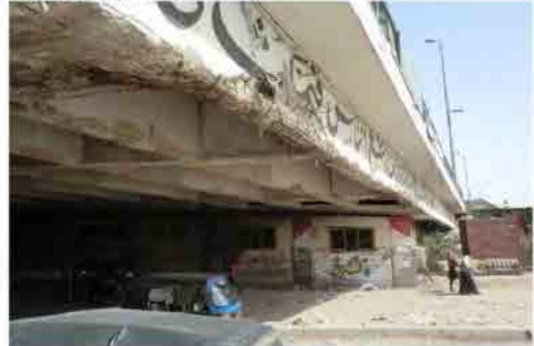
Girder Rebar Exposure (Bad) Severe exposure.
