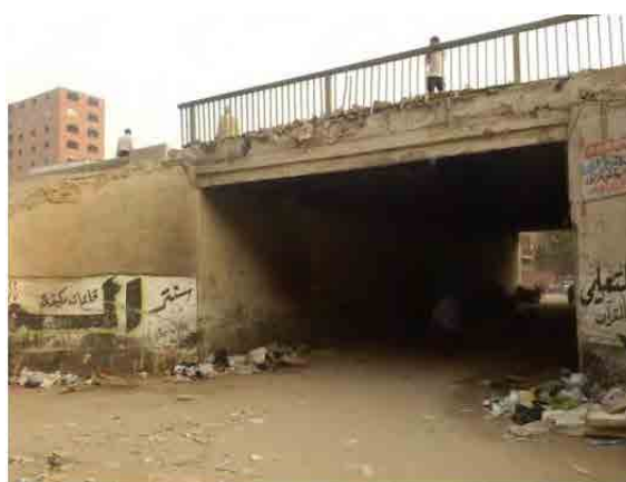
Picture 2-9 Box culvert where repair methods were demonstrated
