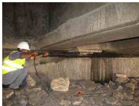
Picture 2-8 Accumulated dirt around a bridge bearing and cleaning with a pressure washer
