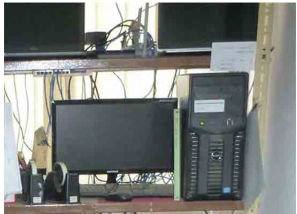
Status of installing the BMS server
