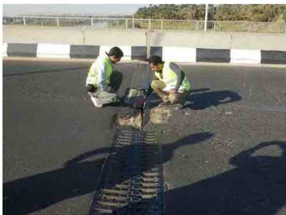
Confirming a faulty expansion device discovered during inspection
