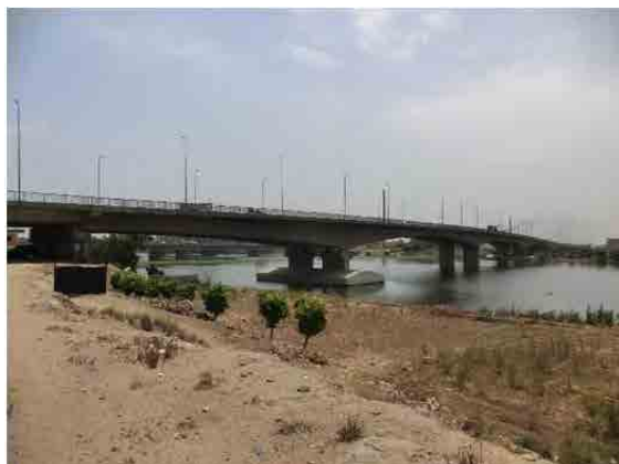
Kafr El-Zayat Bridge
