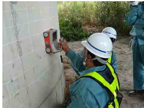
Inspection practice with cover meter
