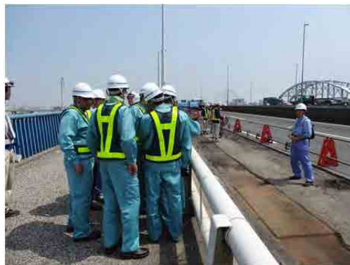
Observation of bridge repair
