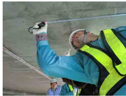
Inspection practice of a concrete bridge
