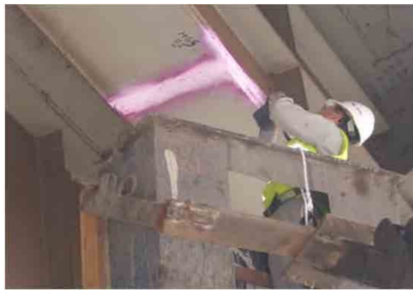
Weld line liquid penetrant inspection
