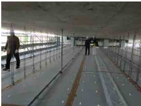
Experience scaffolding for repair work
