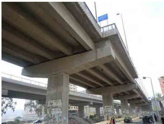
Picture 2-3 Insufficient cleanup at time of construction
