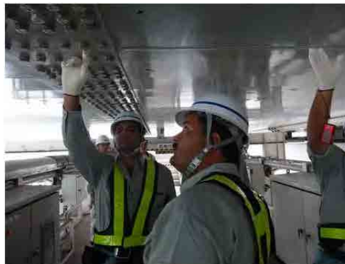
Observation of maintenance of Honshu-Shikoku Bridge
