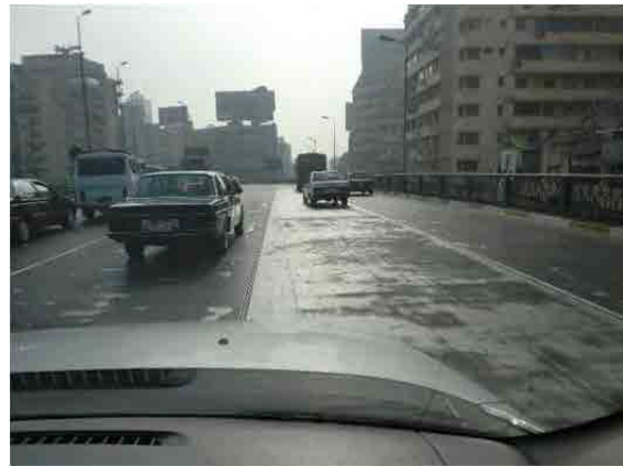
Picture 2-2 Worn-out paving of steel deck
