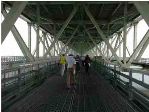
Observation of inspection corridor of Akashi Kaikyo Bridge
