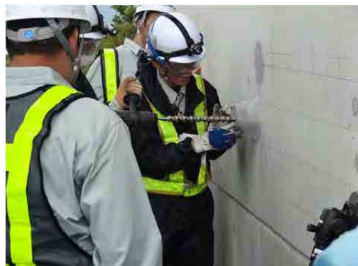
Observation of concrete sampling
