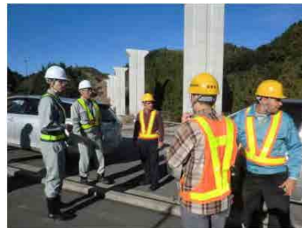
Observation of bridge construction site
