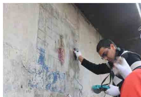
Field Training of Rebar detector (Magnetic type)
