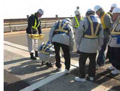
Inspection practice of expansion joint
