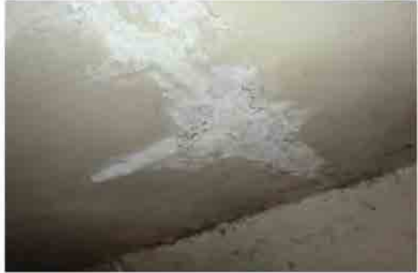
Girder Rebar Exposure (Bad) Severe exposure.
