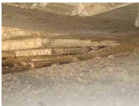
Picture 2-8 Accumulated dirt around a bridge bearing and cleaning with a pressure washer
