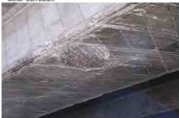
Girder Rebar Exposure (Poor) Minor corrosion.
