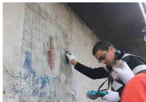
Field Training of Rebar detector (Magnetic type)
