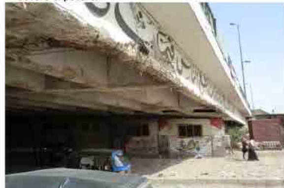
Girder Rebar Exposure (Bad) Severe exposure.
