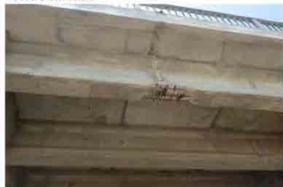
Girder Rebar Corrosion (Bad) Severe corrosion.
