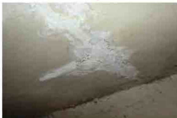
Girder Rebar Exposure (Bad) Severe exposure.
