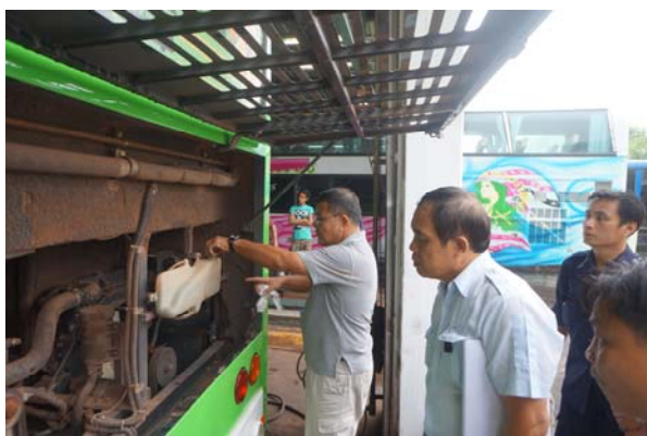
Check Cooling Water
