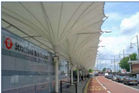
The Project to enhance the capacity of Ventiane capital state bus enterprise May 2012 Public transport facility plan
