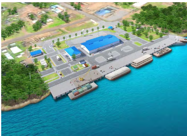
A bird's-eye view of Juba port expansion project
