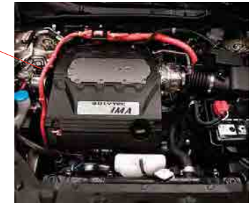
Orange colored wiring
