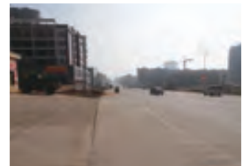
Zhushi-Chengbu Provincial Road
