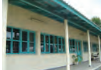
Constructed classroom (CFS* Massinga) * CFS : Training schools for health personnel; mainly at basic level
