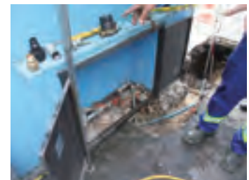
Replacement of water service pipes
