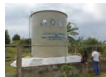
Water supply facility installed in LGU, South Davao Region
