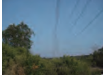
Transmission lines constructed under the project
