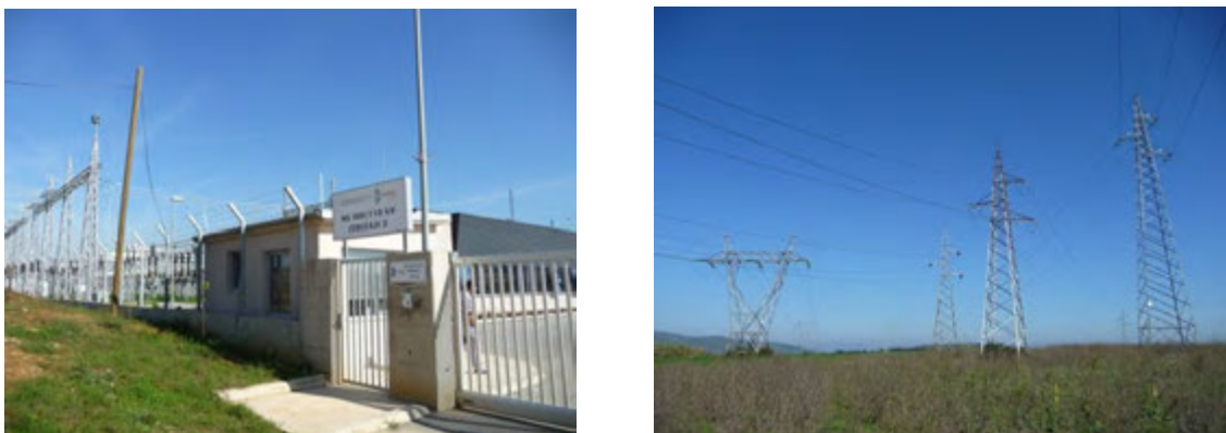
Figure 2-26 Field Verification of Power Lines (Left: Substation, Right: Intercrossing power lines)
