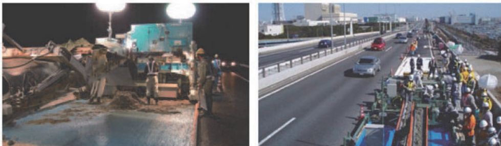
Figure 129 Pictures of implementation of thickening RC slab method
