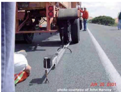
Figure 61 Image of Benkelman Beam Test
