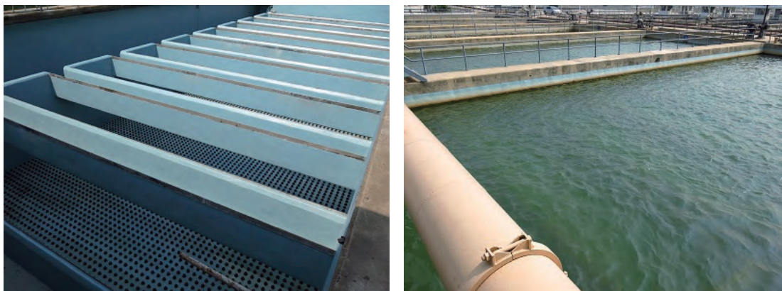
Figure 83 Before and After Repair of Filter Basin
