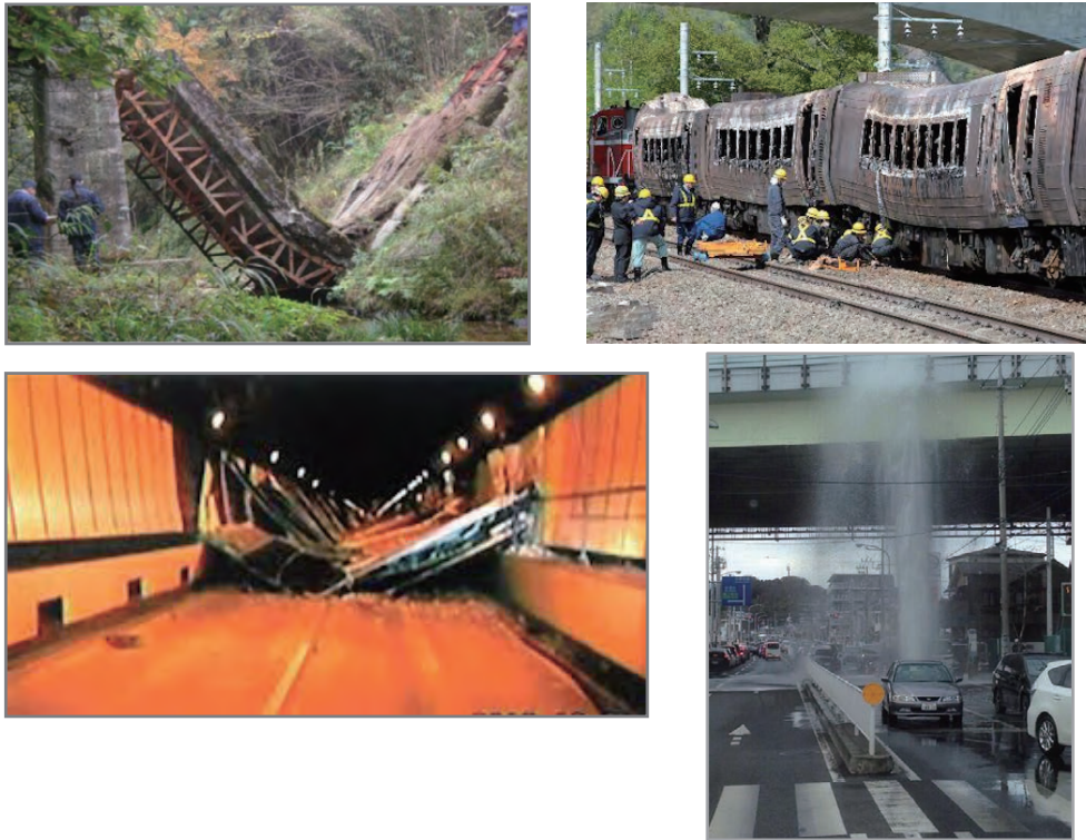
Figure 4 Accidents Caused by Deterioration of a Bridge (above left), a Railway (above right), a Tunnel (below left) and a Water Supply Pipe (below right)
