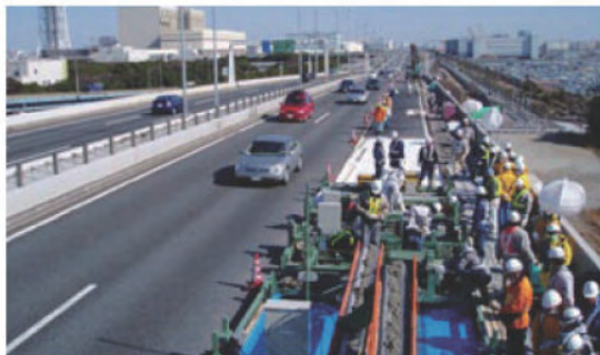
Scene of Placing on Concrete Slab of an Elevated Bridge
