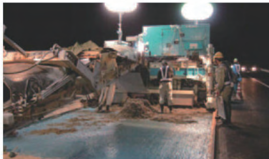
Scene of Placing on Concrete Slab of an Elevated Bridge
