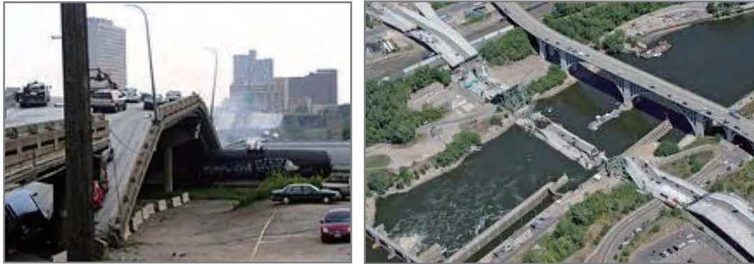
Figure 25 Scene of the Collapse of the Highway Bridge in Minneapolis
