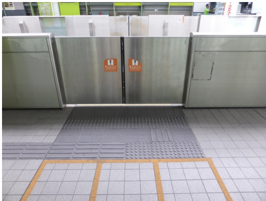
Platform door (closed)
