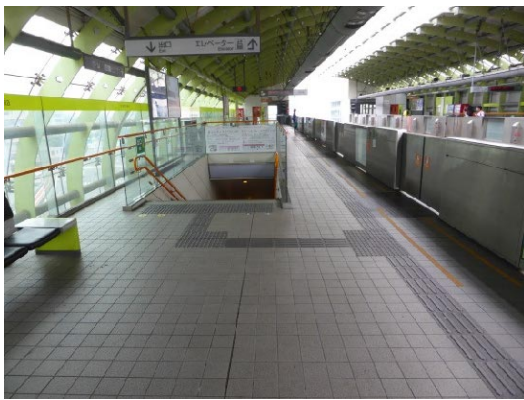
Stairs on platform
