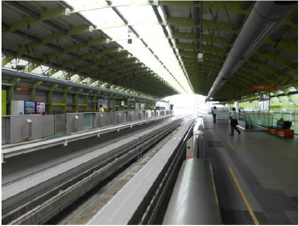
Figure 5.3.14 Separate Platform Type (Tama Monorail Japan)
