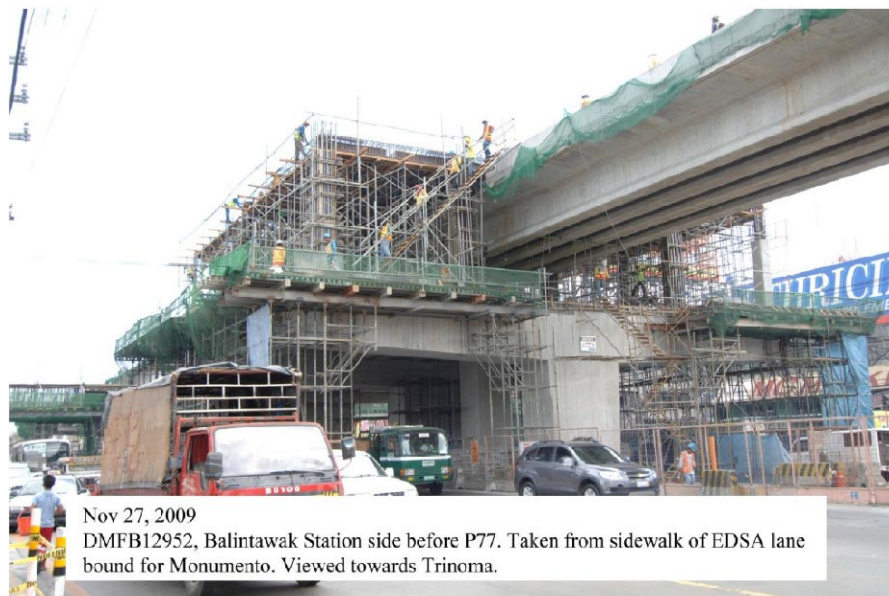
Figure 5.3.39 Station Cantilever Pier Construction (Sample)
