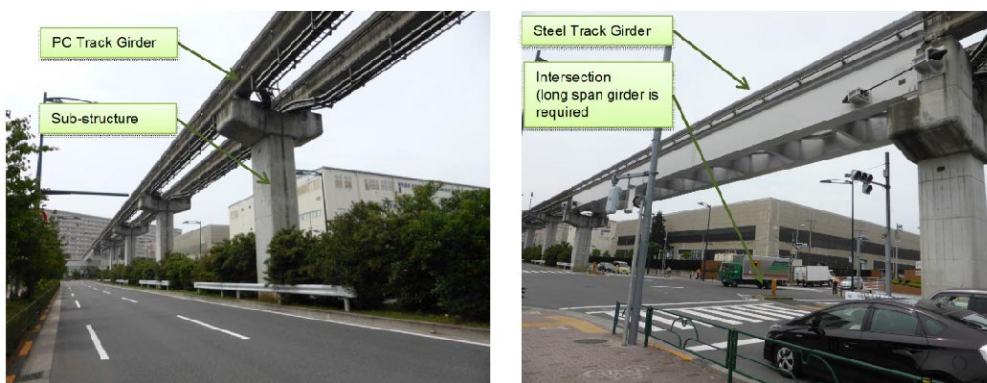
Figure 5.3.6 PC Track Girders with Mono-type Piers.
