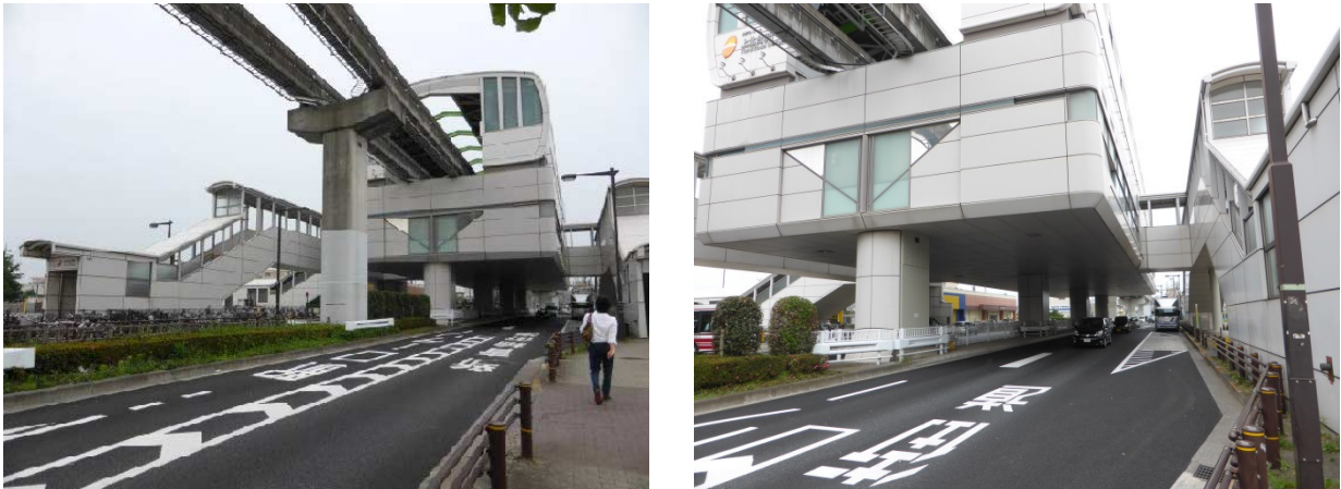
Figure 5.3.21 Station Building with Single Central Piers (Tama Monorail Japan)
