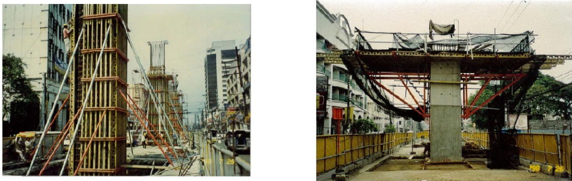
Figure 5.3.33 Pier Column Construction (Manila)
