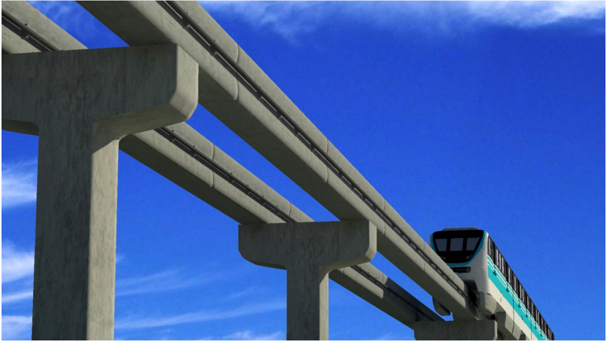
Images of Monorail Rolling Stocks and Civil Structures
