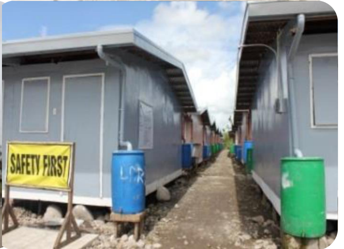
Figure 9.5-12 Bunkhouses at Brgy. Tacuranga
