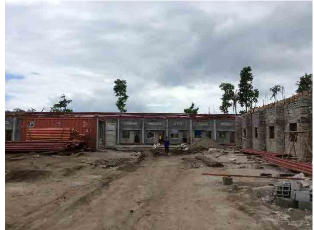
Figure 9.5-24 Resettlement Housing Under Construction in Barangay Sacme
