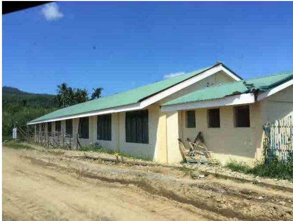
Figure 9.5-8 School in Tacloban North
