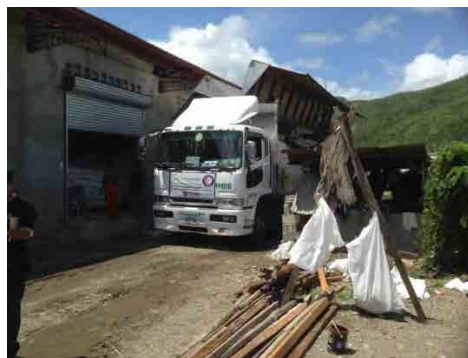
Extension warehouse near the DSWD HUB
