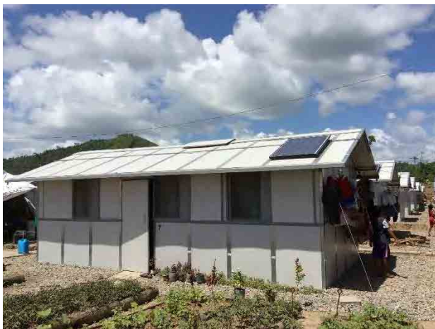
Figure 9.5-13 Transitional Shelters by Tsu Chi Foundation in BRG. San Jose
