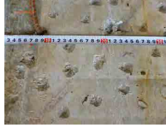
Photo 22. This chipping photo is column of using ready mixed concrete site.
