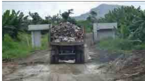
Debris being transported
