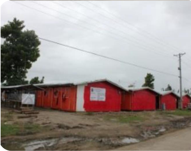
Figure 9.5-11 Bunkhouses at Brgy. Candahug
