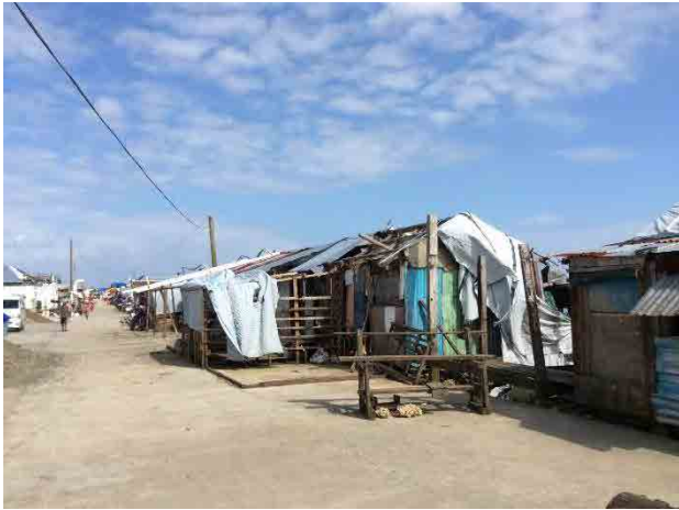
Figure 9.5-27 Informal Settlement in a Coastal Barangay
