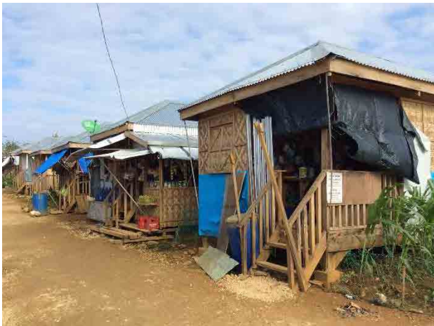
Figure 9.5-29 Temporary Shelters in Barangay Cogon
