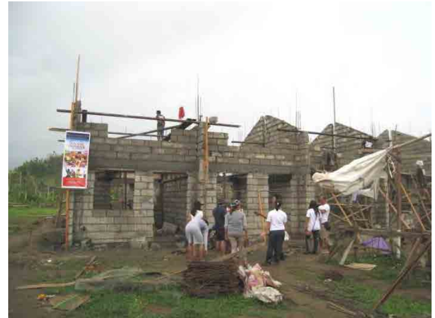
Figure 9.5-20 Resettlement Housing Under Construction in Barangay Pago, as of May 2014
