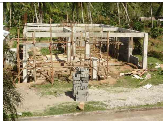
Coconut tissue culture laboratory under construction, NCRC-V, Baybay city, Leyte
