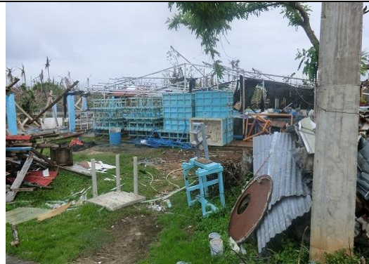
Damaged Cultivating Tank
