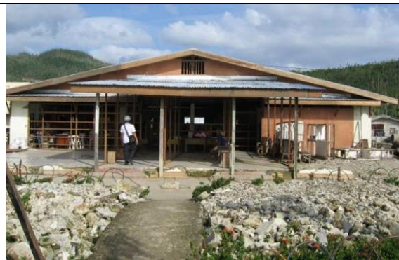
Before Typhoon, this office has 2nd floor with Reinforced Concrete(Marabut)
