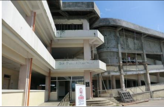
Damage by Storm Surge on 1 st Floor of EVRMC
