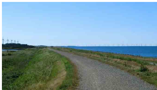
Figure 2.2-30 Example of Tidal Embankment with Greenery Revetment (The Lolland Island in Denmark)
