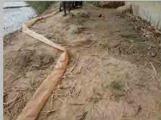
No. 4 Condition of road surface
