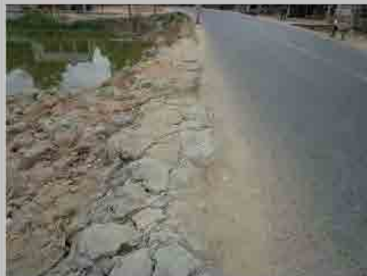
No. 3 Distance view to the forward left
