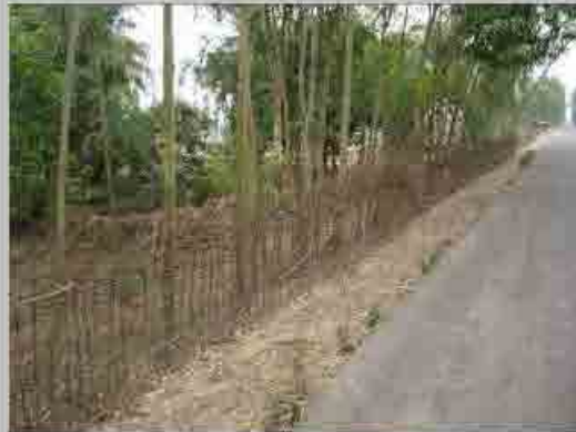
No. 3 Distance view to the forward left
