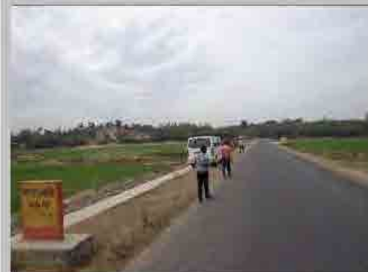
No. 3 Distance view to the forward left
