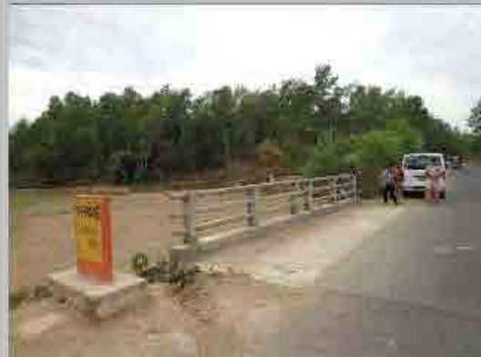
No. 3 Distance view to the forward left
