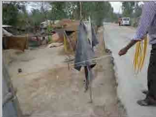
No. 3 Distance view to the forward left
