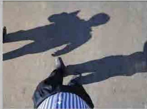
No. 4 Condition of road surface
