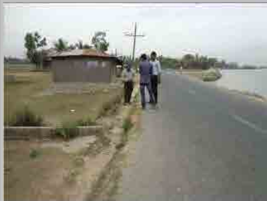
No. 3 Distance view to the forward left
