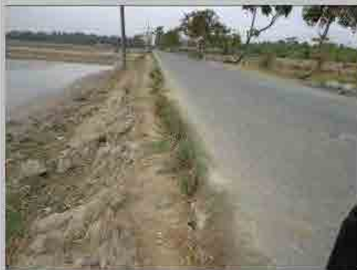
No. 3 Distance view to the forward left
