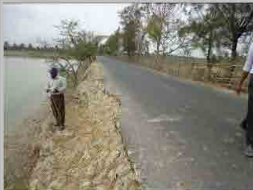
No. 3 Distance view to the forward left
