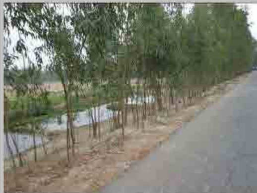
No. 3 Distance view to the forward left
