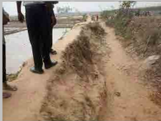
No. 3 Distance view to the forward left
