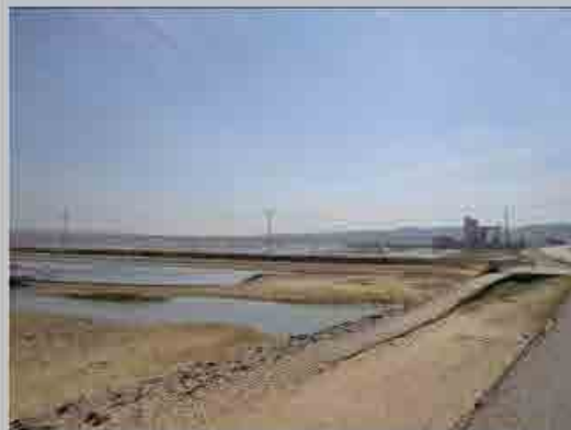
No. 3 Distance view to the forward left
