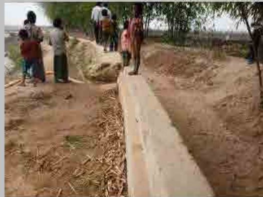
No. 3 Distance view to the forward left
