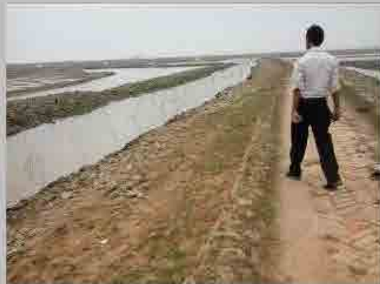
No. 3 Distance view to the forward left
