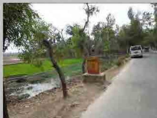
No. 3 Distance view to the forward left
