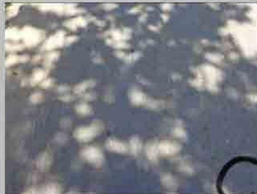
No. 4 Condition of road surface
