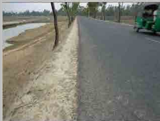
No. 3 Distance view to the forward left
