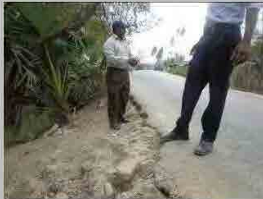
No. 3 Distance view to the forward left
