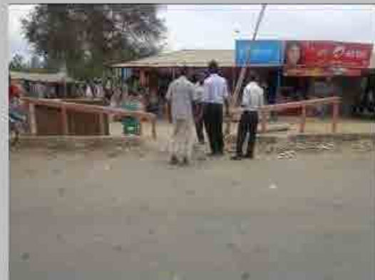
No. 4 Condition of road surface
