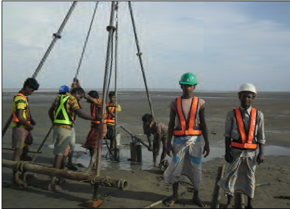
Figure -1 Soil boring at Matarbari site
