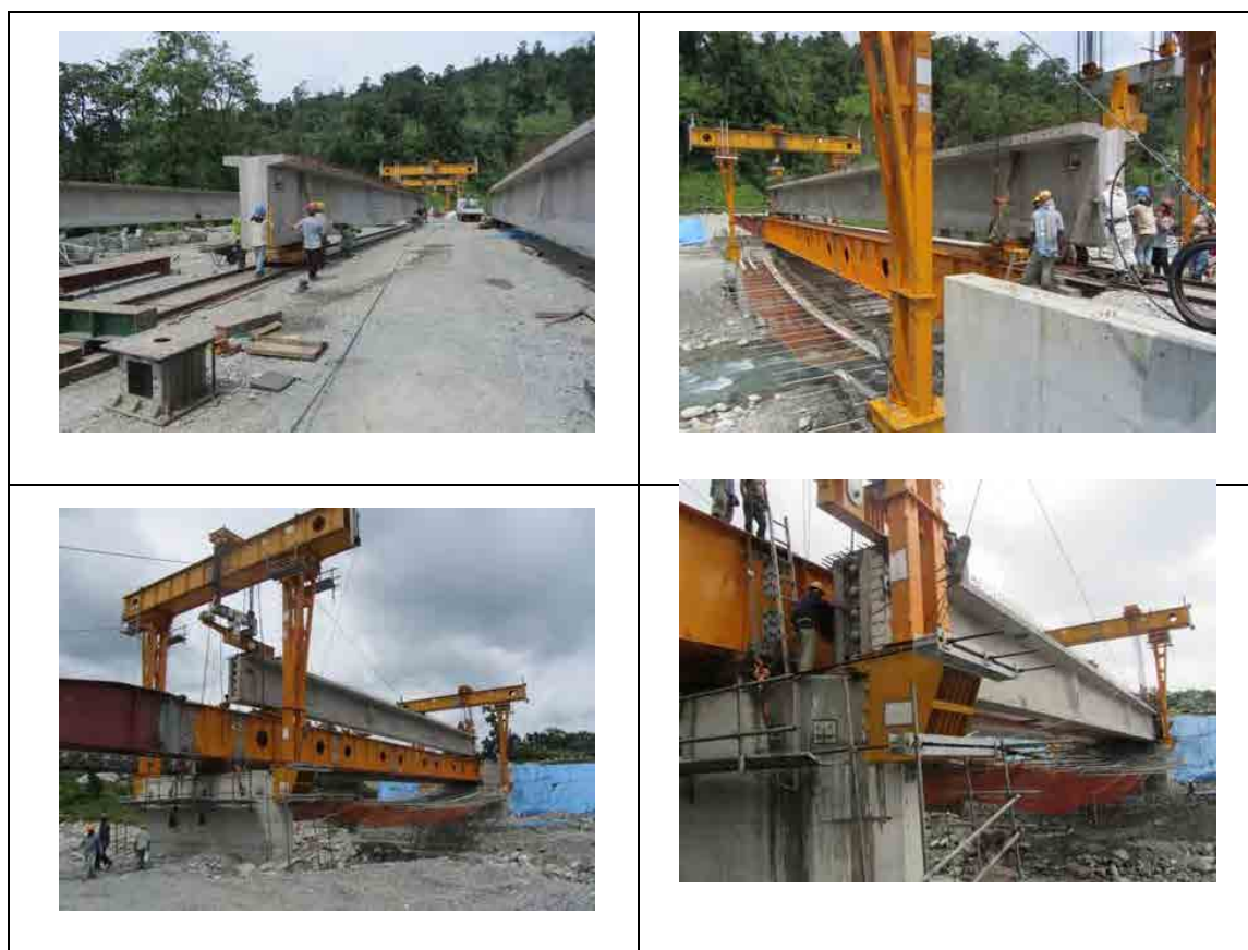
Figure 16.4-9 Reference Pictures of Erection Girder Method
