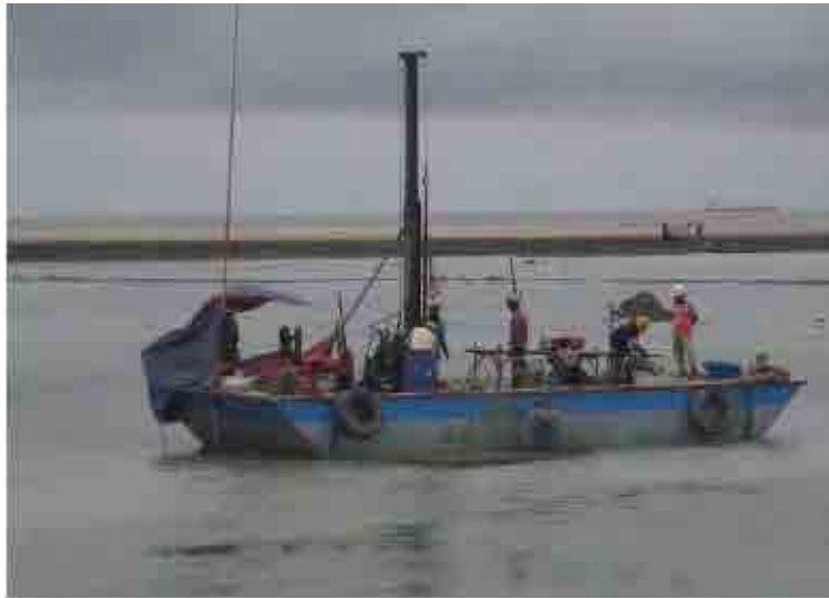
Figure 17.3-1 Floating Stage for the Shallow Water Drilling
