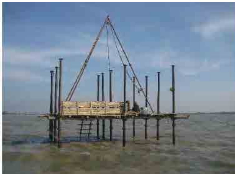
Figure 17.3-3 Stationary Platform for Drilling
