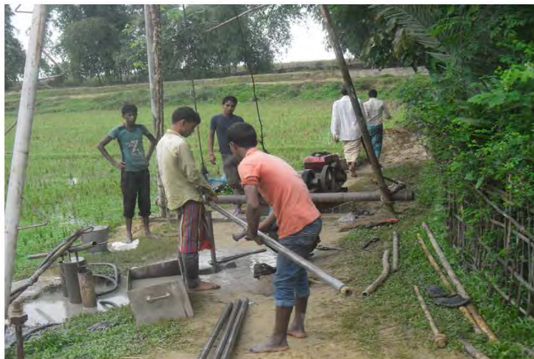
Photograph for BH: Existing Box-2
