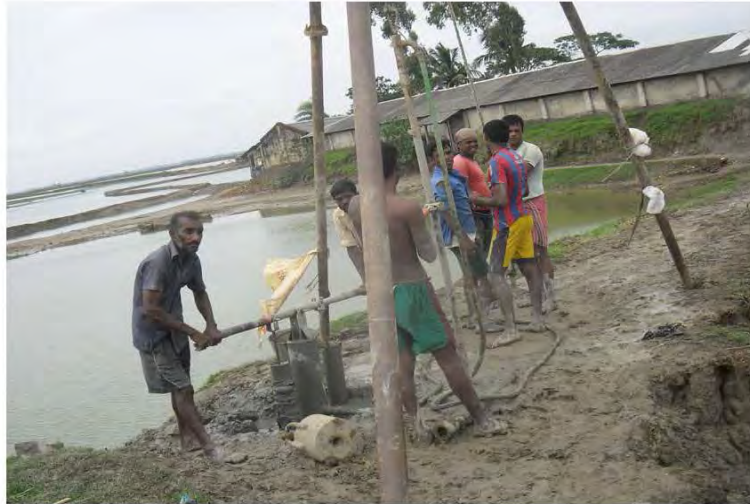
Photograph for BH: Existing Box-3
