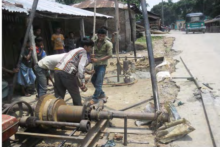
Photograph for BH: Existing Box-1
